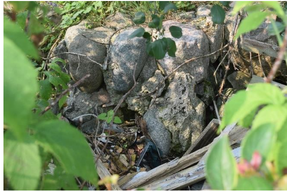
Plate 30: Remaining stone foundation, looking southwest
