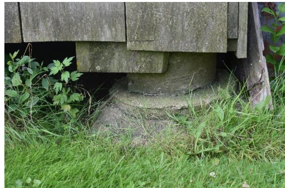
Plate 28: Concrete footing, looking south
