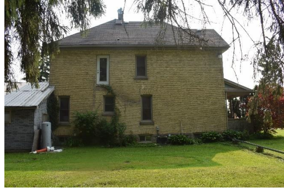
Plate 26: West elevation, looking east
