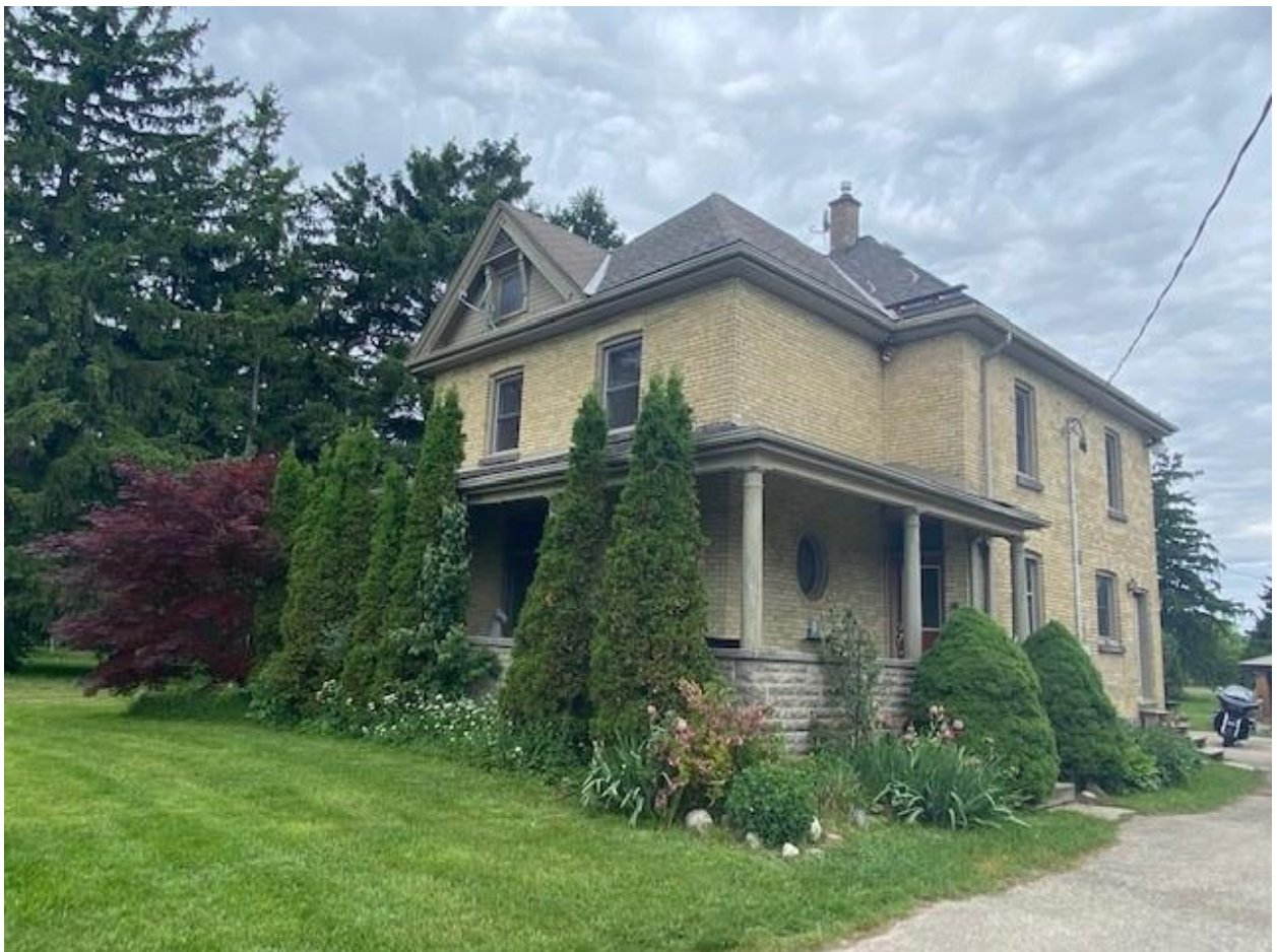
Image 2: South-east elevations of house on property showing wrap-around veranda and hip roof
