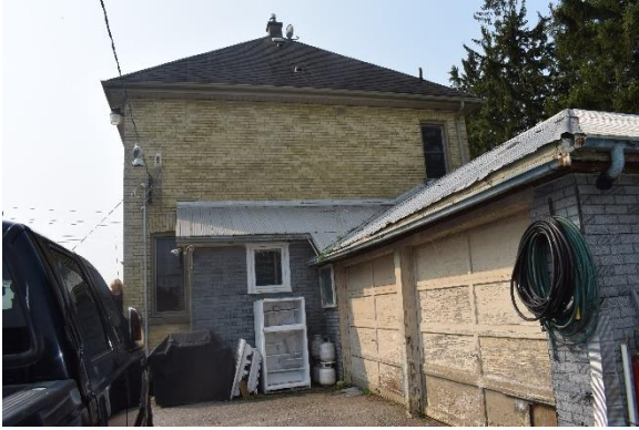
Plate 25: Additions, looking south
