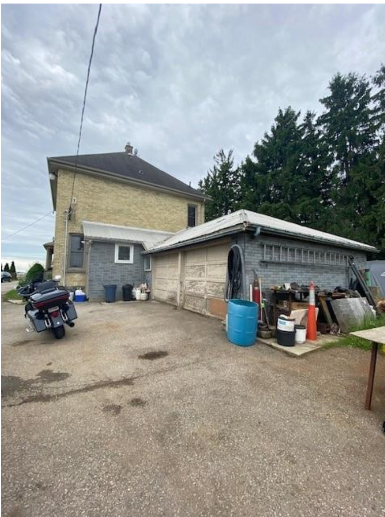
Image 6: Rear, north elevation of house on property showing contemporary garage additions and added rear entrance
