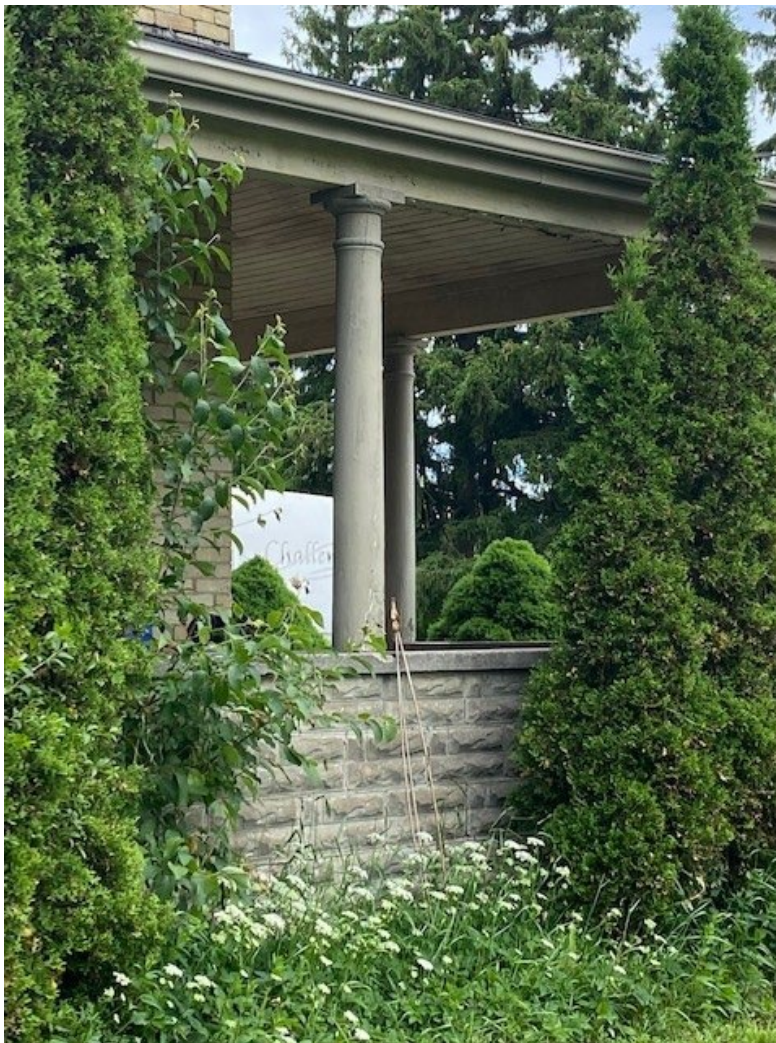
Image 14: Porch details showing wood columns with concrete block surround
