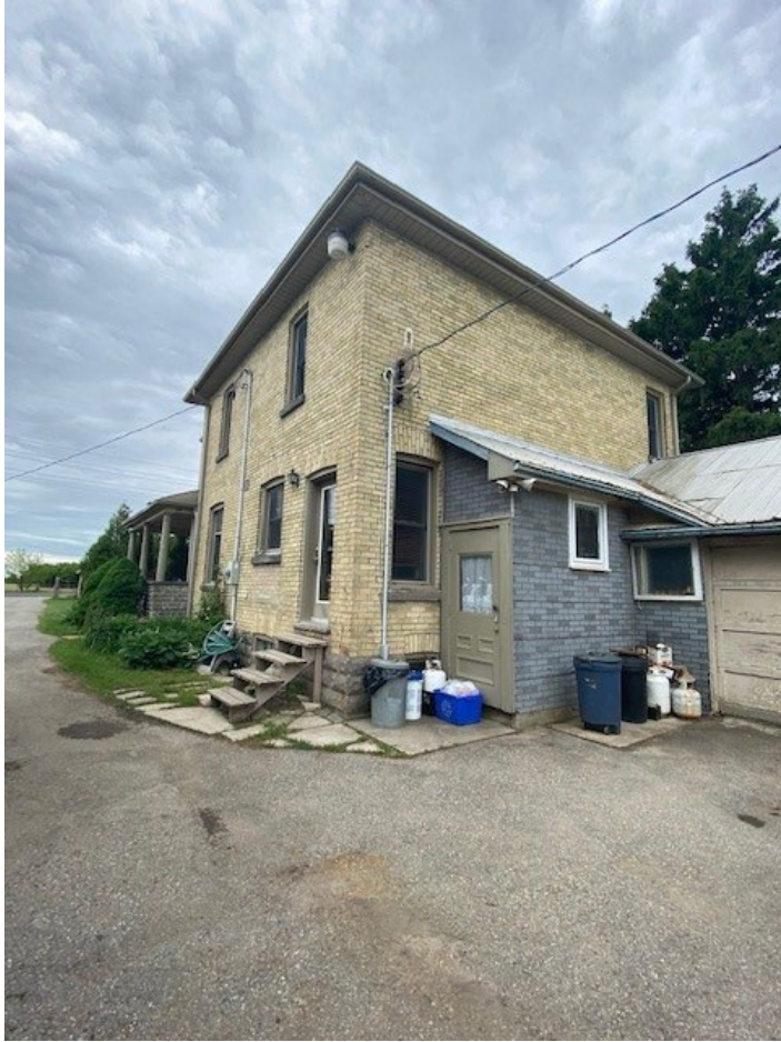
Image 7: North-east elevations of house on property showing rear entrance addition
