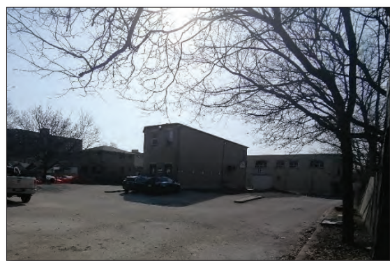
Figure 31: North (rear) elevation looking south-east (MHBC, 2022).
