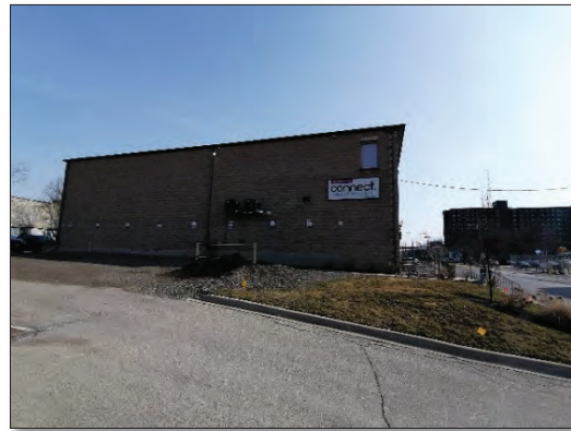
Figure 29: West elevation looking eastward (MHBC, 2022).
