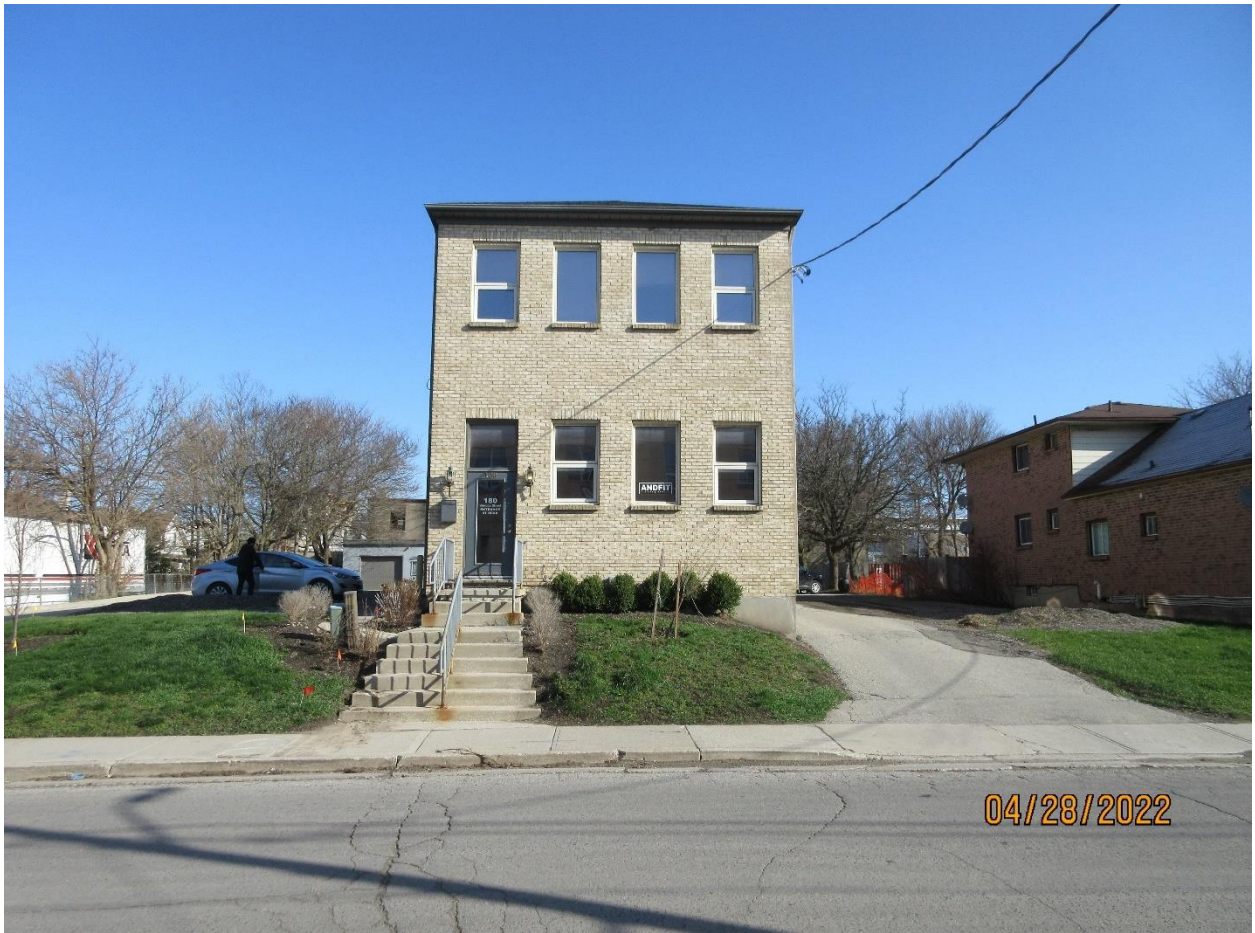
Image 2: View of the front façade of the property at 180 Simcoe Street.
