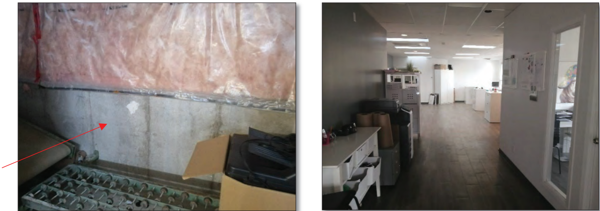
Figures 32 & 33: (left) View of poured concrete foundation in basement; (right) View of interior of second floor (MHBC, 2022).
