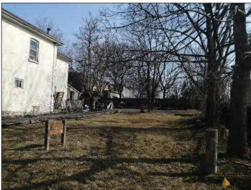
Figure 38: View of south elevation and rear yard of property (MHBC, 2022)
