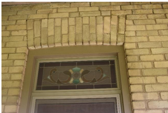
Plate 20: Stained glass transom, looking north
