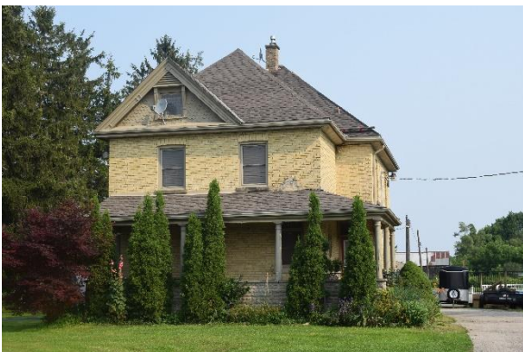
Plate 15: Looking north showing two and one half storey structure, hip roof, brick chimney, gable dormer, and projecting east bay
