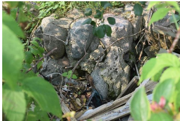
Plate 30: Remaining stone foundation, looking southwest
