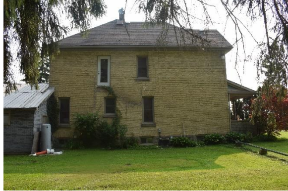
Plate 26: West elevation, looking east
