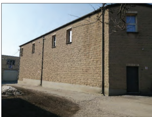
Figure 30: East elevation looking west from north-east corner of property (MHBC, 2022).
