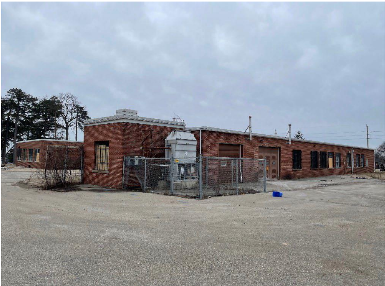
Figure 10. Building #2 (B12150) Ontario Government Building, facing north-east – Zelinka, Mar 2022
