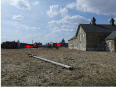
31.7m (104 ft) to south structure demolition activity.
