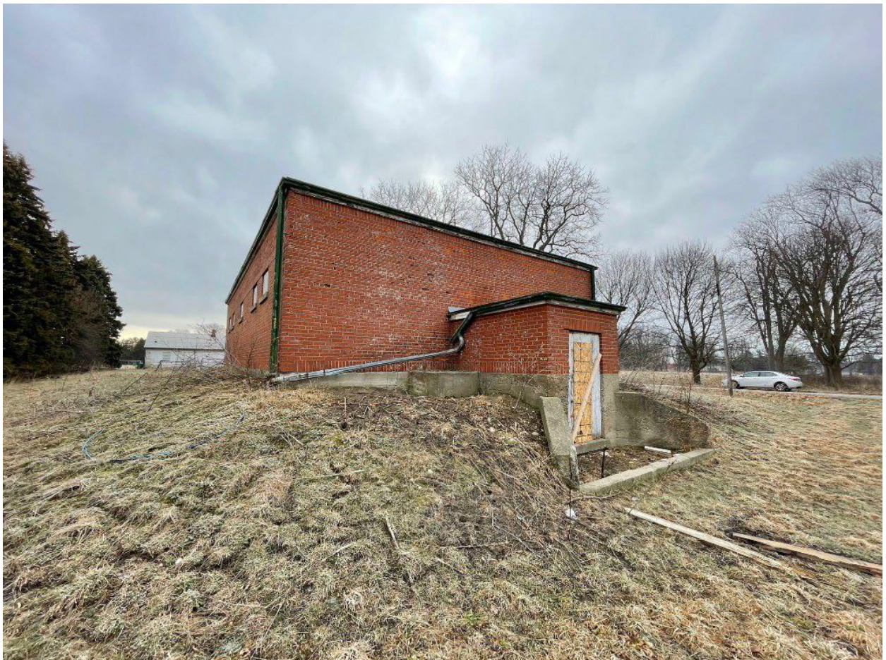
Figure 16. Building #4 (B12016) Granary, facing east – Zelinka, Mar 2022
