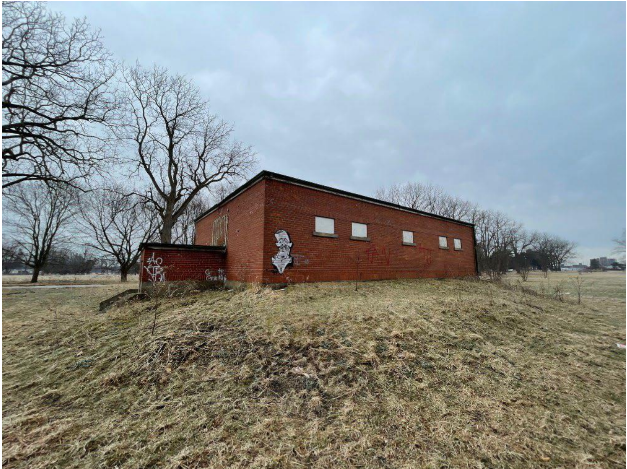
Figure 18. Building #4 (B12016) Granary, facing south-west – Zelinka, Mar 2022
