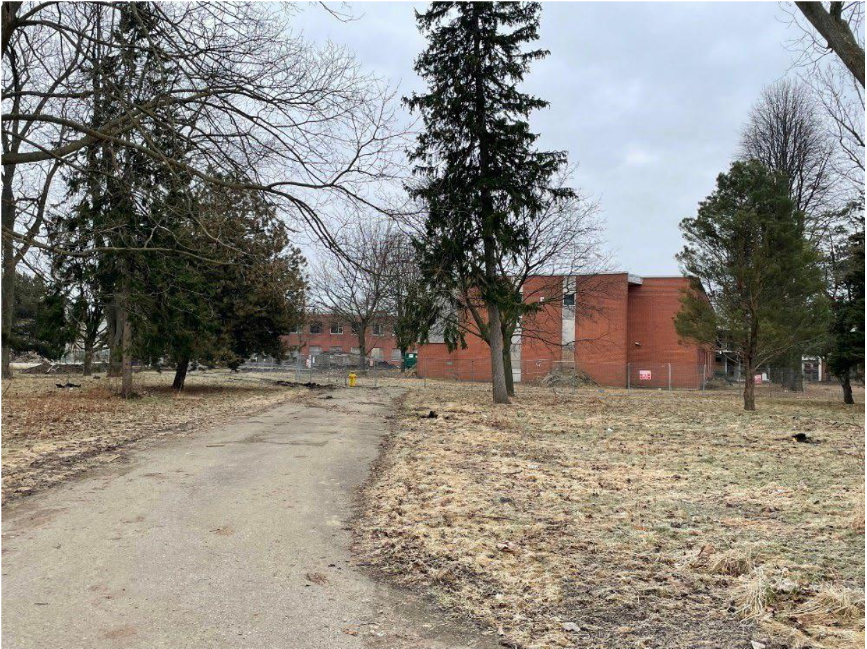
Figure 3. Building #1 (B12013) North Pavilion Building, facing south-east – Zelinka, Mar 2022
