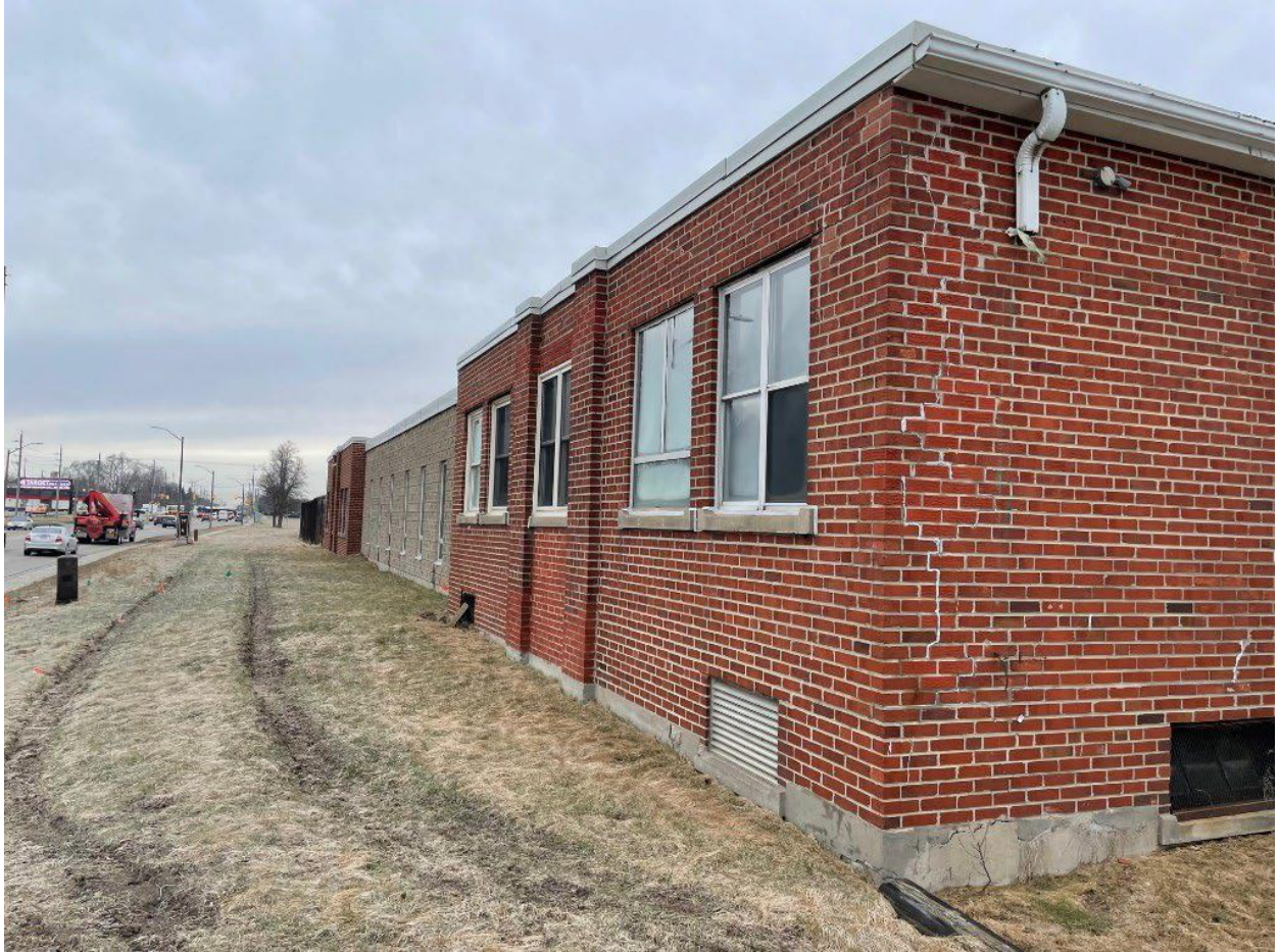
Figure 9. Building #2 (B12150) Ontario Government Building, facing north-east – Zelinka, Mar 2022
