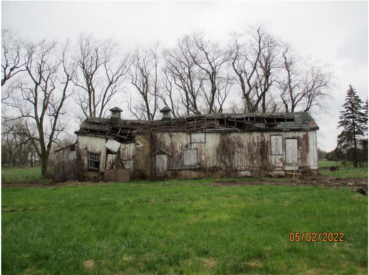
Figure 23. Building #6 (B17057) Potting Shed, facing north – M. Greguol, May 2022
