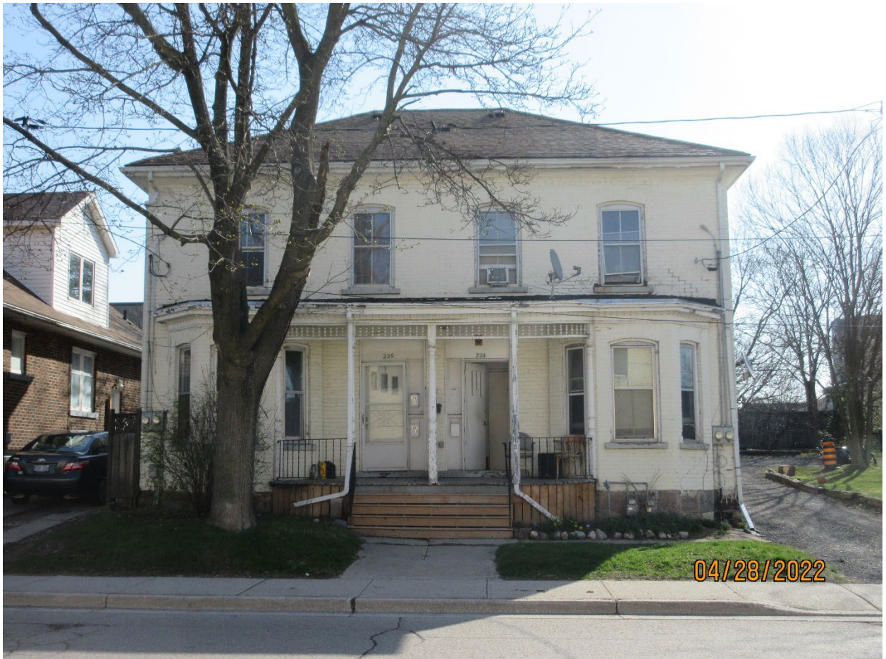
Image 6: Photograph of the heritage designated property at 224-226 Richmond Street.
