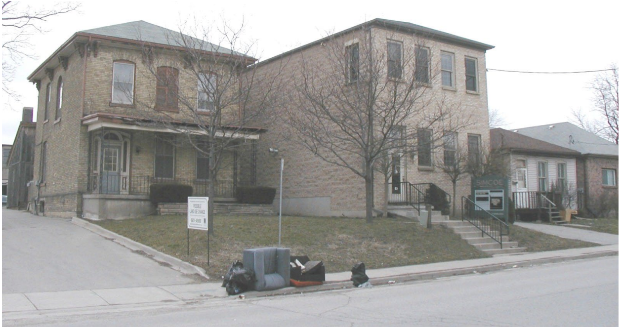
Image 5: View of the properties at 178 Simcoe Street (left), 180 Simcoe Street, and 182 Simcoe Street in 2002. The buildings on 178 Simcoe Street and 182 Simcoe Street were demolished in 2002.
