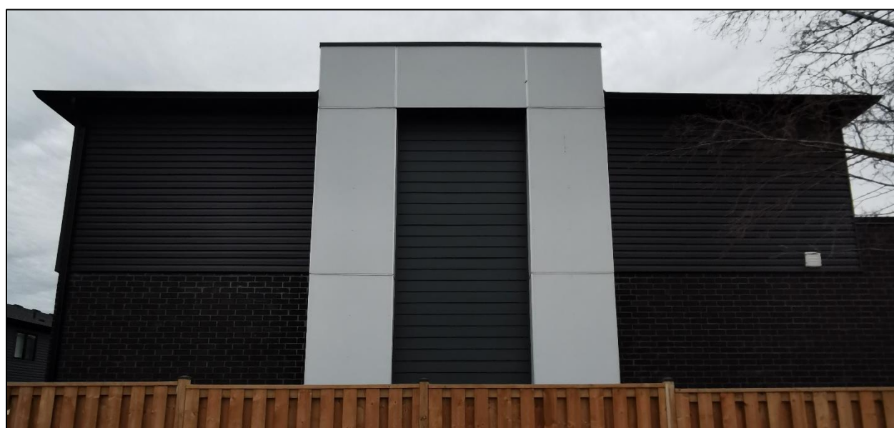
Figure 7. View of 499 Sophia Crescent – Unit 30, Facing East Towards the Subject Lands (2021)
