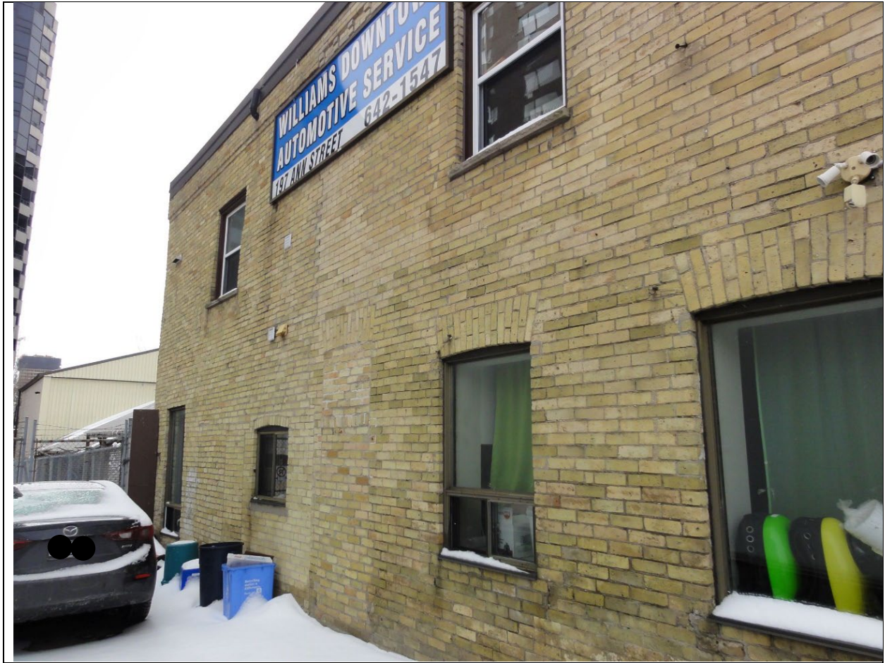
Image 3: East side exterior view of primary building
