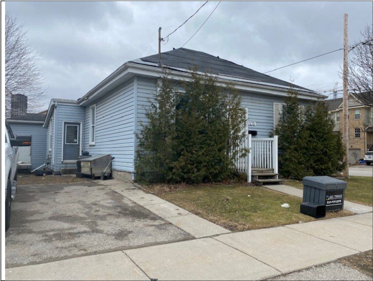
Image 24: 175 Ann Street – view of front and partial side elevation, facing southwest (L.E.Dent, Apr 1, 2022)
