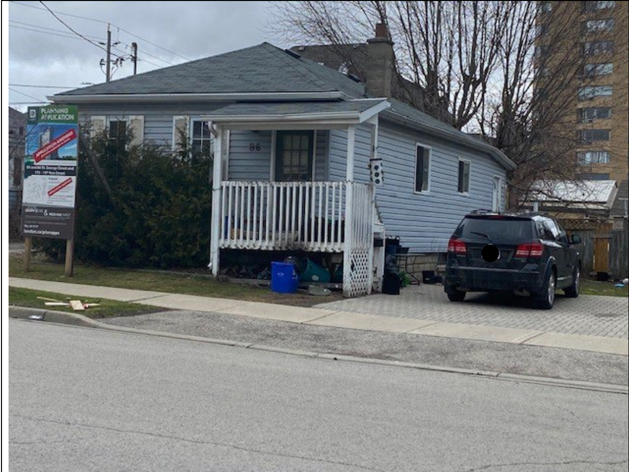
Image 26: 86 St. George Street – view of front and partial side elevation, facing northwest (L.E.Dent, Apr 1, 2022)
