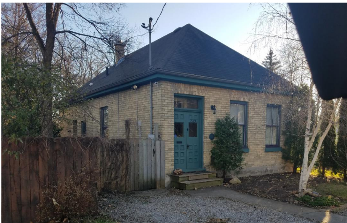
8. 239 Hill Street looking south
