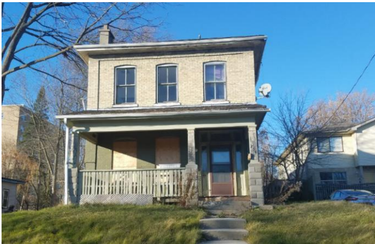
7. 254 Hill Street looking north
