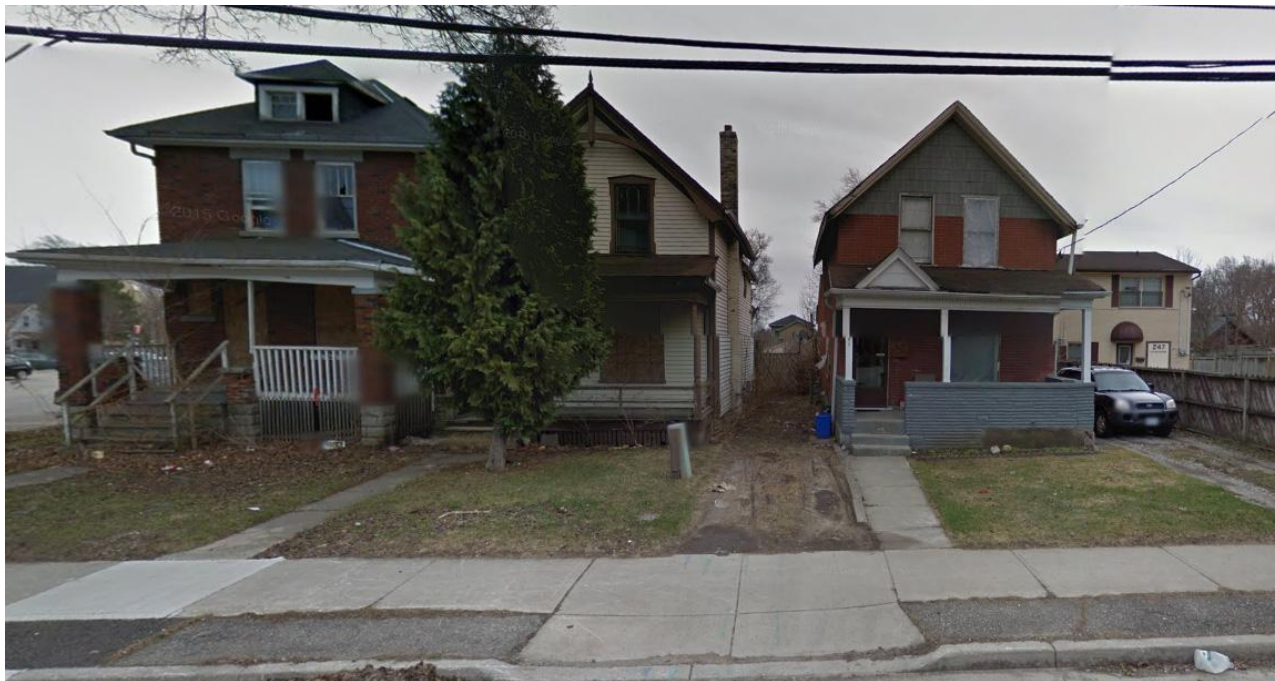
4. Single detached homes on Grey Street in the east portion of the subject lands. To be demolished.
