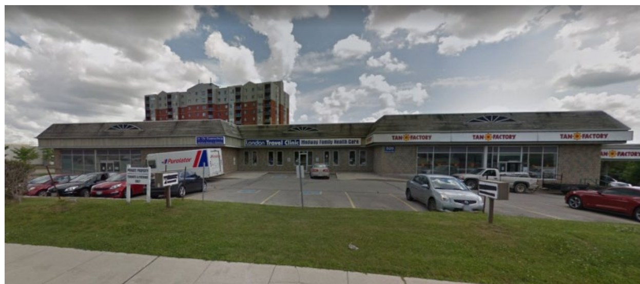
Figure 1 – Existing Commercial Building
