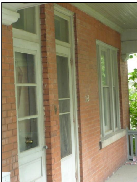
368 Central Window Sill Detail
