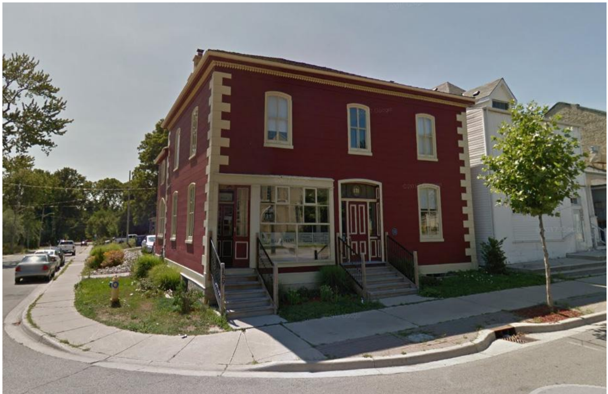
5. 129, 131 Wellington Street looking west
