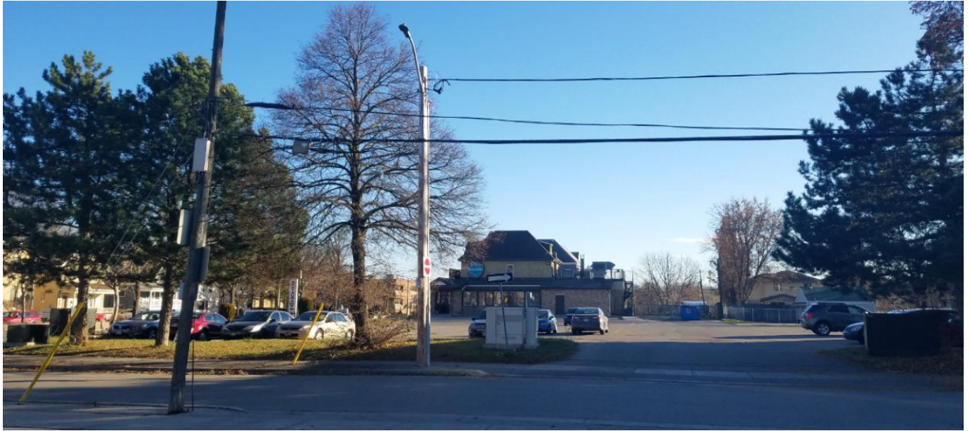
1. Subject lands from Grey street, looking south
