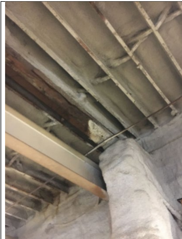
Image 9: Interior view of underside of old washhouse roof and wall
