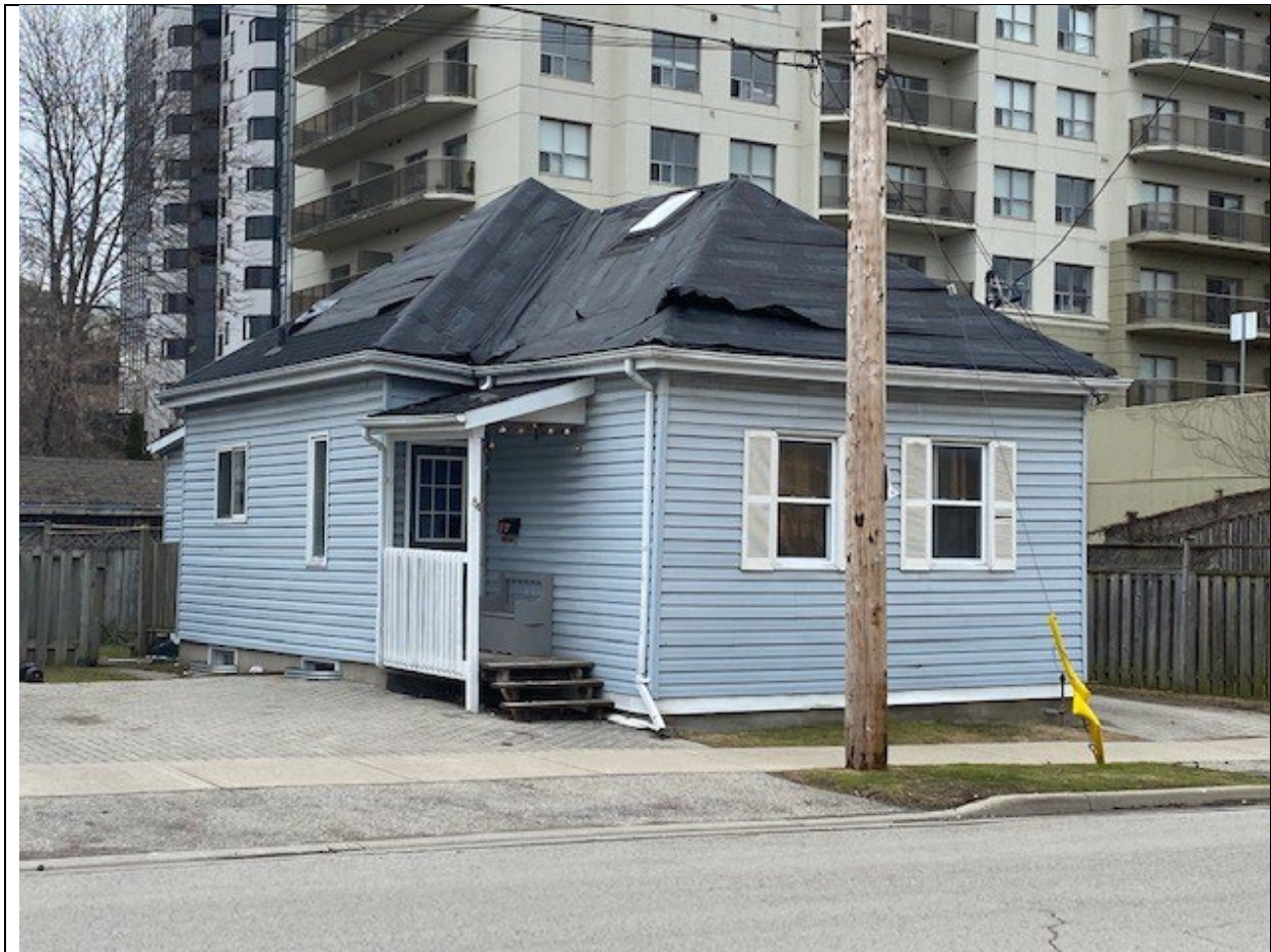
Image 27: 84 St. George Street – view of front and side elevation, facing southeast (L.E.Dent, Apr 1, 2022)
