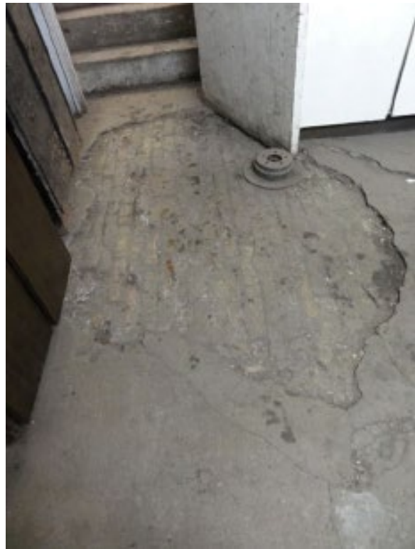
Image 6: Detail of partially exposed original brick floor – primary building
