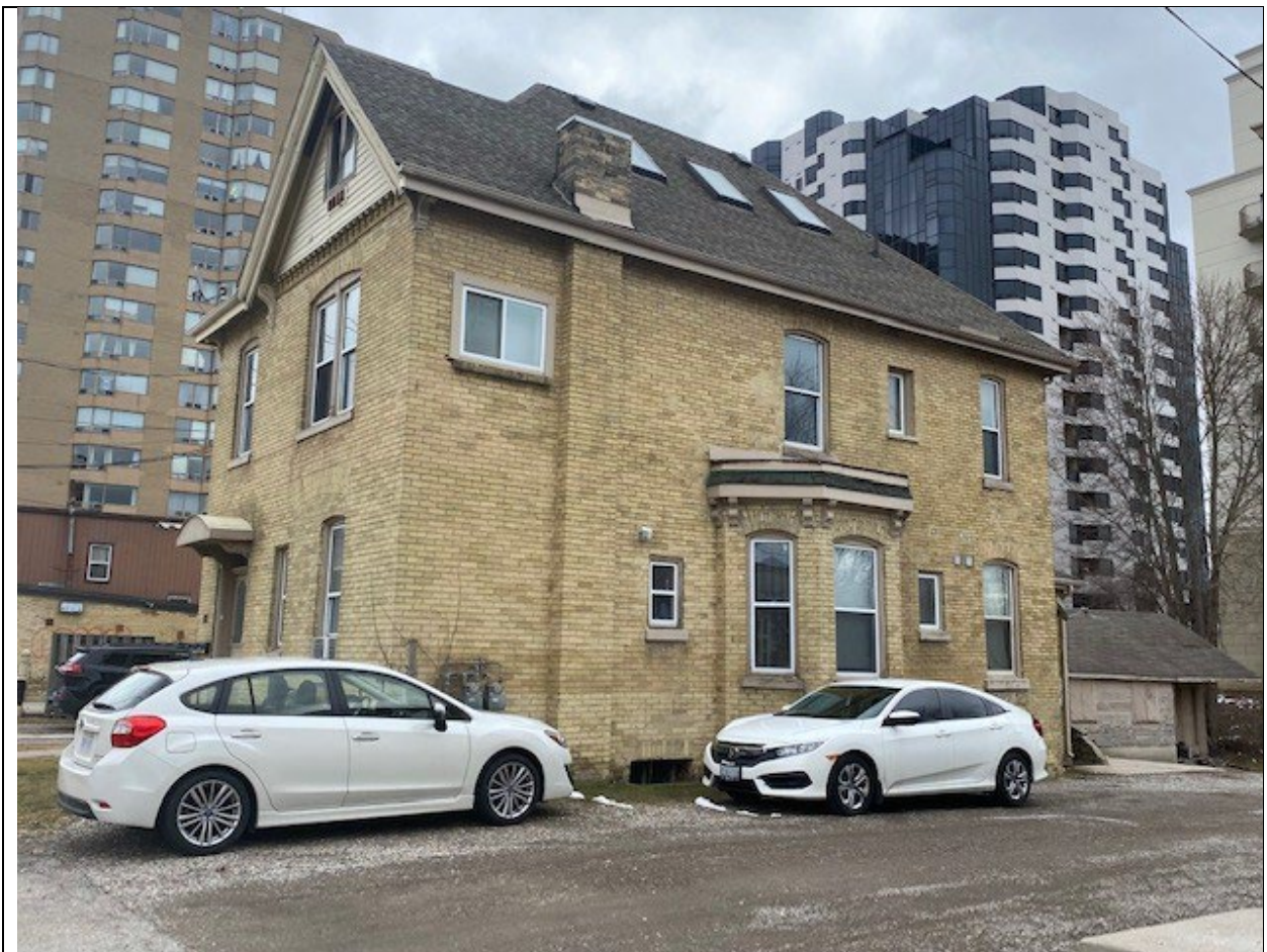
Image 19: 183 Ann Street – view of side and partial front elevation, facing southeast (L.E.Dent, Apr 1, 2022)
