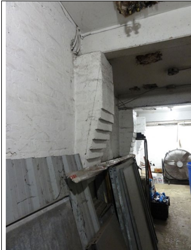
Image 5: Stacked corbelled brick support – primary building basement
