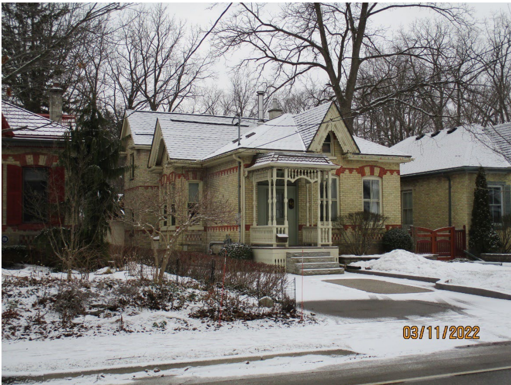
Image 14: Photograph of the dwelling located at 41 Bruce Street showing a two-storey gable-roof addition added to the rear of the dwelling located at 41 Bruce Street. The side-hall plan cottage form of this property is clearly articulated through the massing of the building, and the addition at the rear is distinguishable from the original dwelling. The use of the roof shapes and forms help to minimize the visibility of the addition from street (2022).
