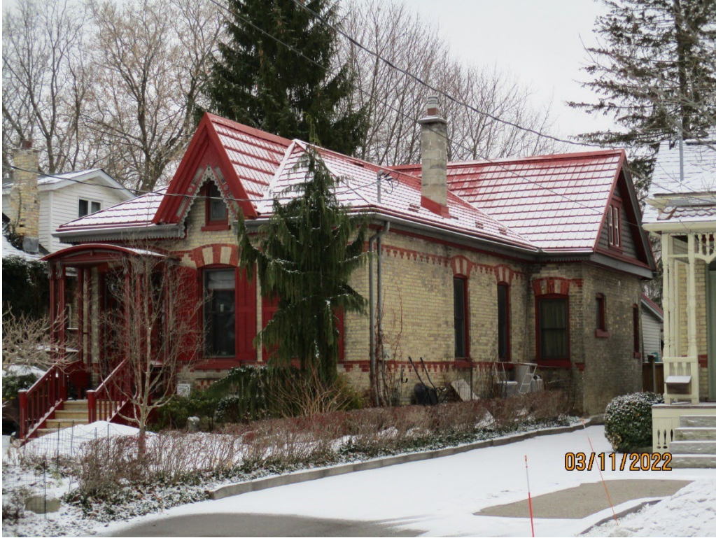
Image 13: Photograph of the dwelling located at 43 Bruce Street showing a rear addition to the existing single storey cottage. In this compatible addition, the use of a cross-gable has been used to minimize the visibility of the increase in building height at the rear of the dwelling (2022).
