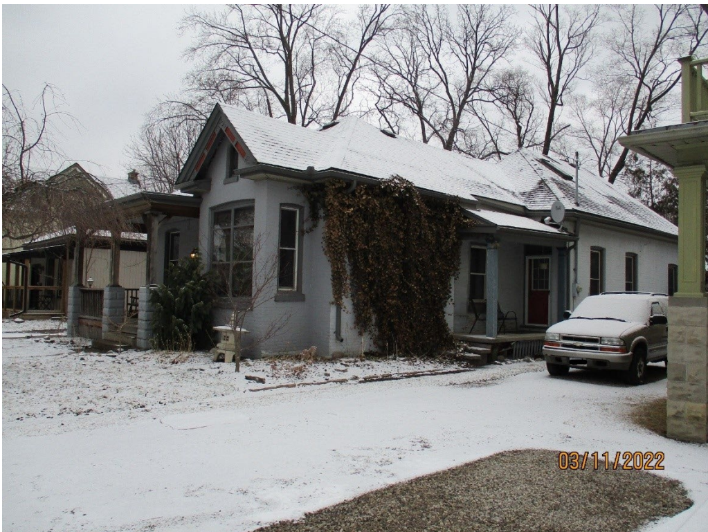
Image 16: Photograph of the dwelling at 44 Byron Avenue East showing a rear addition added to the existing one storey dwelling while also maintaining the scale, form, and mass of the single storey dwelling. In this example, a modest addition has been added to the rear of the cottage to add additional living space to the dwelling (2022).
