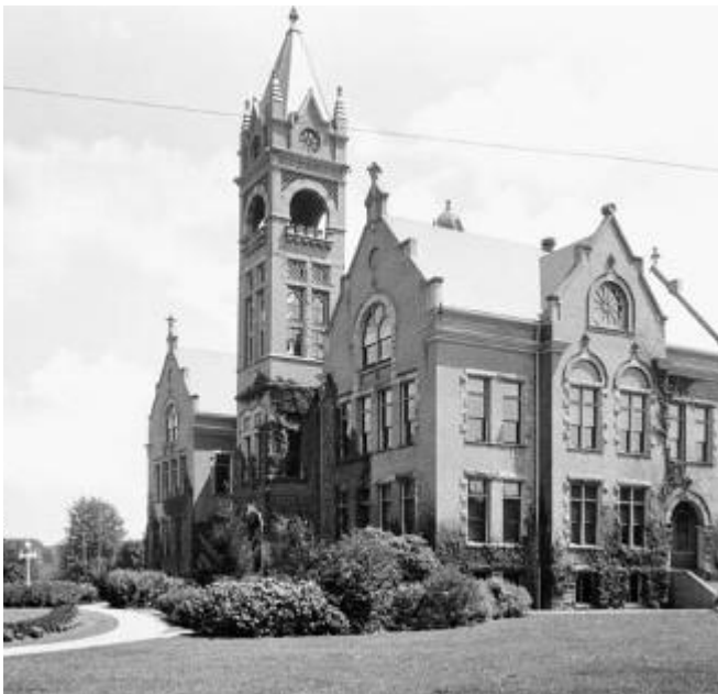
Image 5: Views of the London Normal School from Wortley Road Circa 1920. The LNS is located just southeast of Wortley Road and the main village along Elmwood Ave. Source: Canada's Historic Places. London Normal School. https://www.historicplaces.ca/en/rep-reg/place-lieu.aspx?id=8871 . Retrieved 2021.
