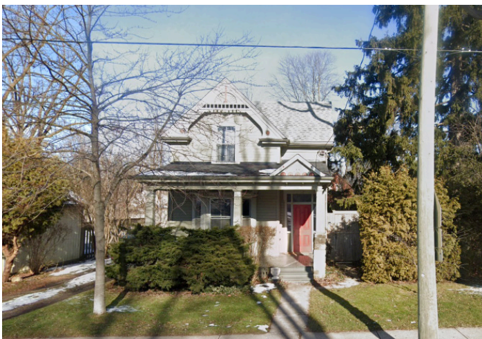
Image 13: 22 Byron Ave. E., South Elevation. Google Streetview, 2021.
