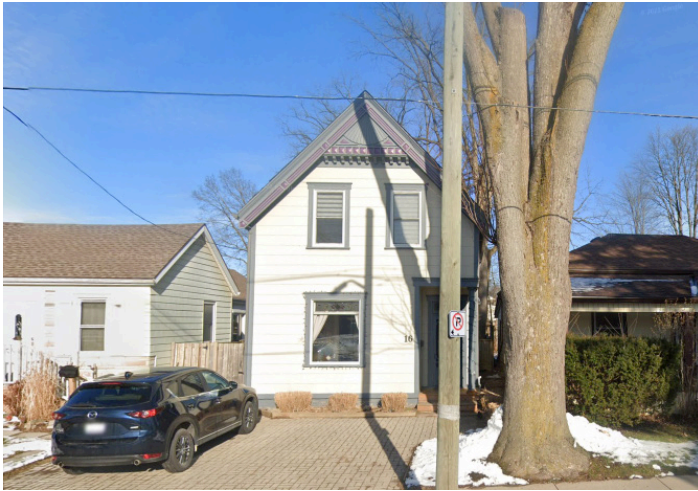
Image 12: 16 Byron Ave E. South Elevation. Google Streetview, 2021.
