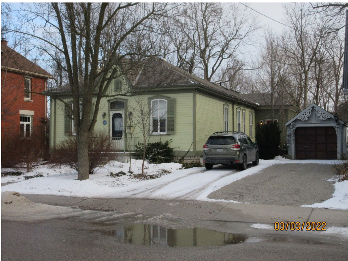
Image 18: 139 Briscoe Street East, a Part IV designated property with a compatible rear addition. In this example, the cottage form and type has been retained in its entirety and the addition has been added to the rear. Its location at the rear of the historic dwelling and its difference in colour helps to distinguish the original dwelling from the addition. The addition is clearly subordinate to the existing dwelling (2022).
