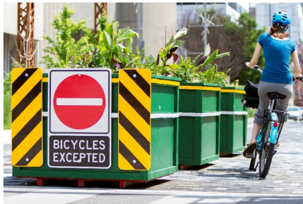
Traffic changes on Dundas Place to support safety and mobility for all during core construction – example of bike detour signs to help cyclists navigate construction safely
