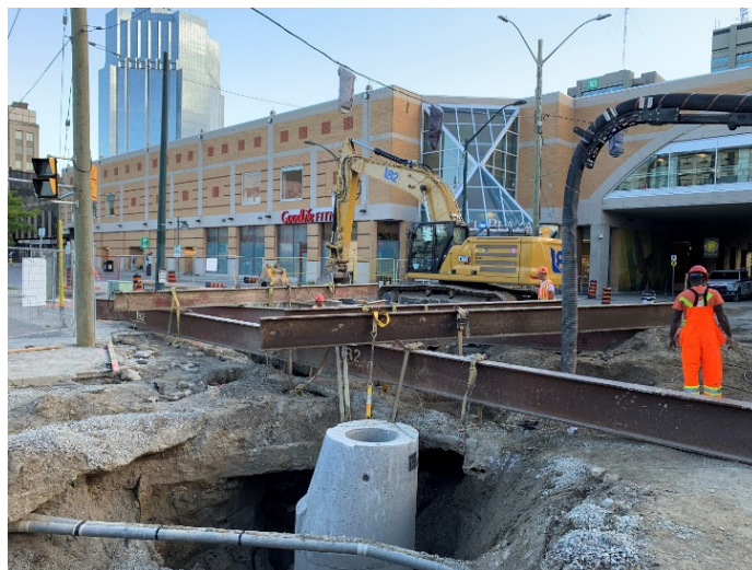
New maintenance hole structure supported by multiple beams at Clarence and King intersection
