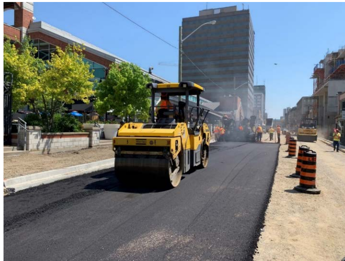
Paving top surface on King Street between Talbot and Richmond Streets.
