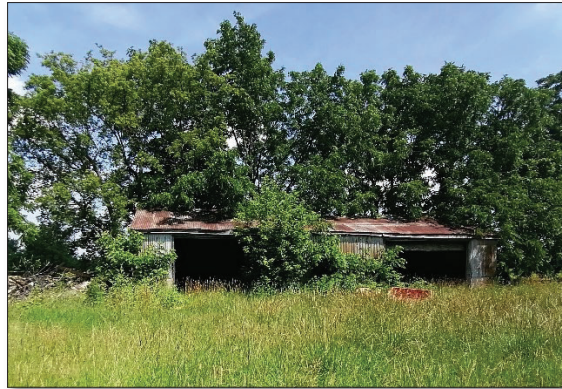
Figure 26: View of outbuilding 3 looking north (MHBC, 2021)
