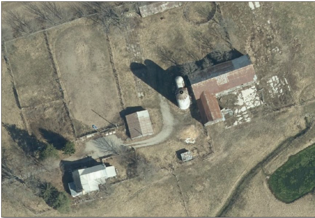
Figures 1 & 2: (above) View of the subject property outlined by red (MHBC, 2021); (below) Aerial photograph of 3700 Colonel Talbot Road, City of London (VuMap, 2021).
