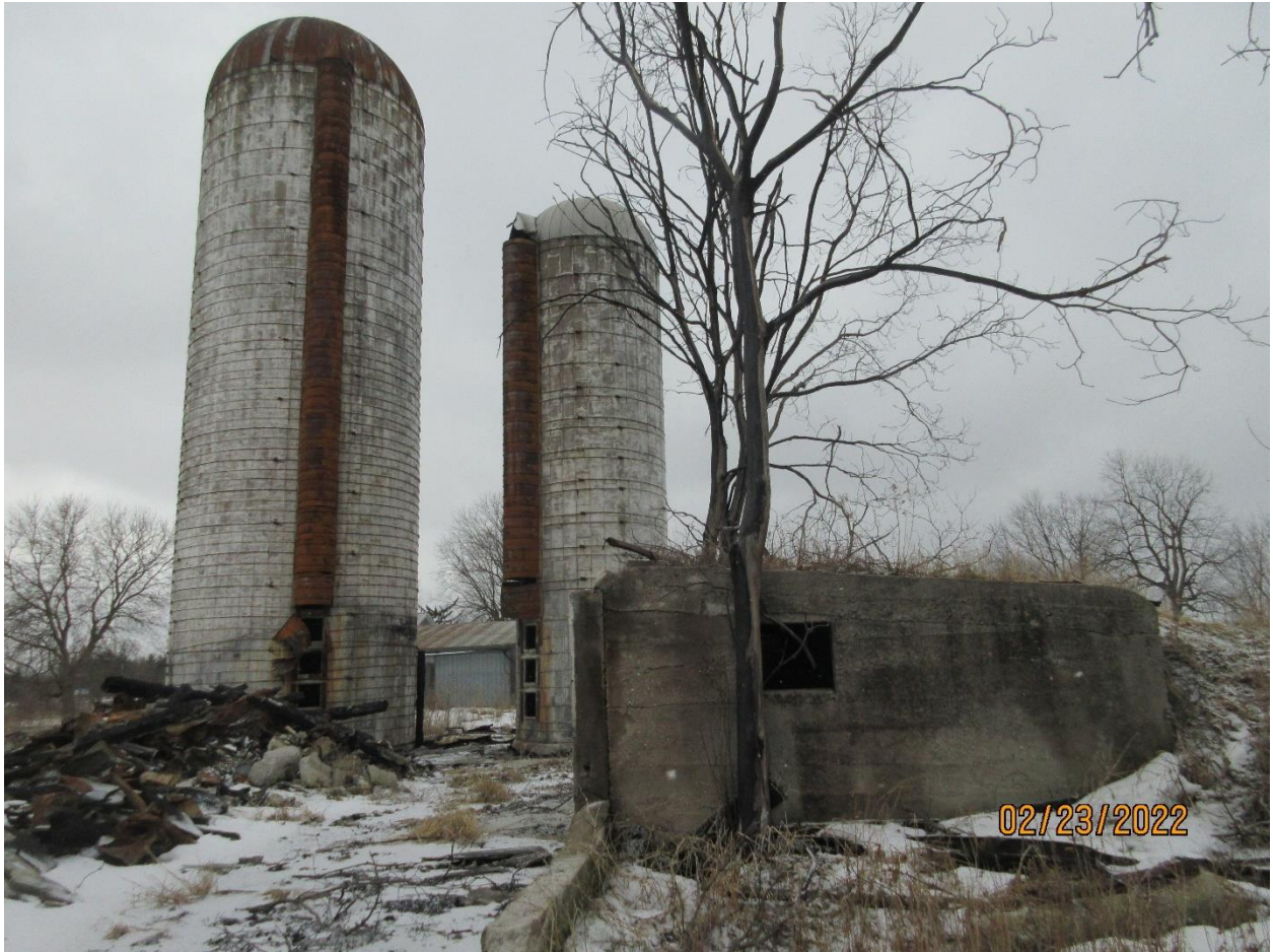
Image 15: View of the silos, showing one of the concrete gangways (barn hill).
