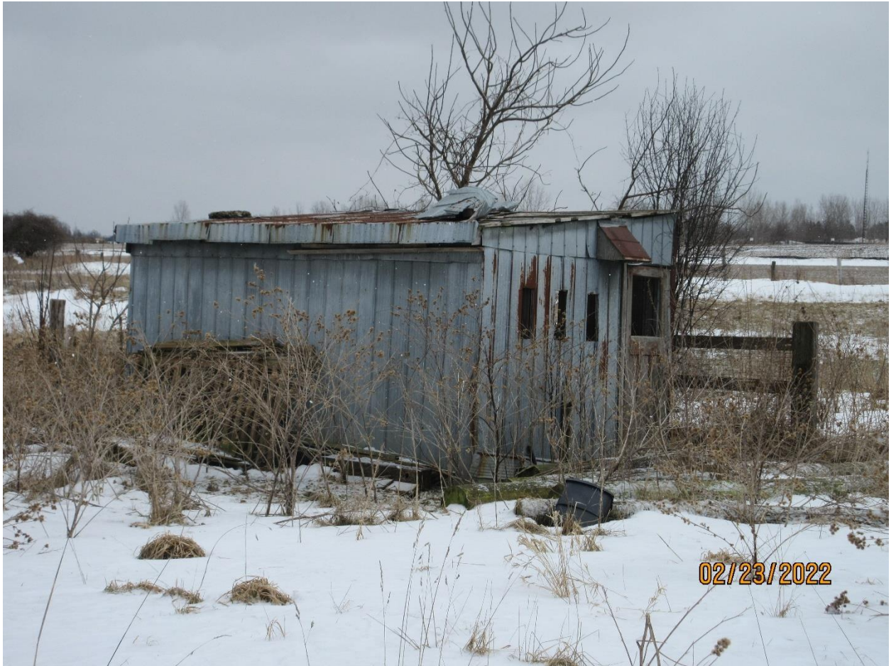
Image 13: View of the shed at 3700 Colonel Talbot Road.
