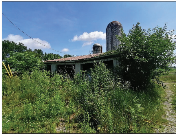
Figure 25: View of outbuilding 2 looking east (MHBC, 2021)
