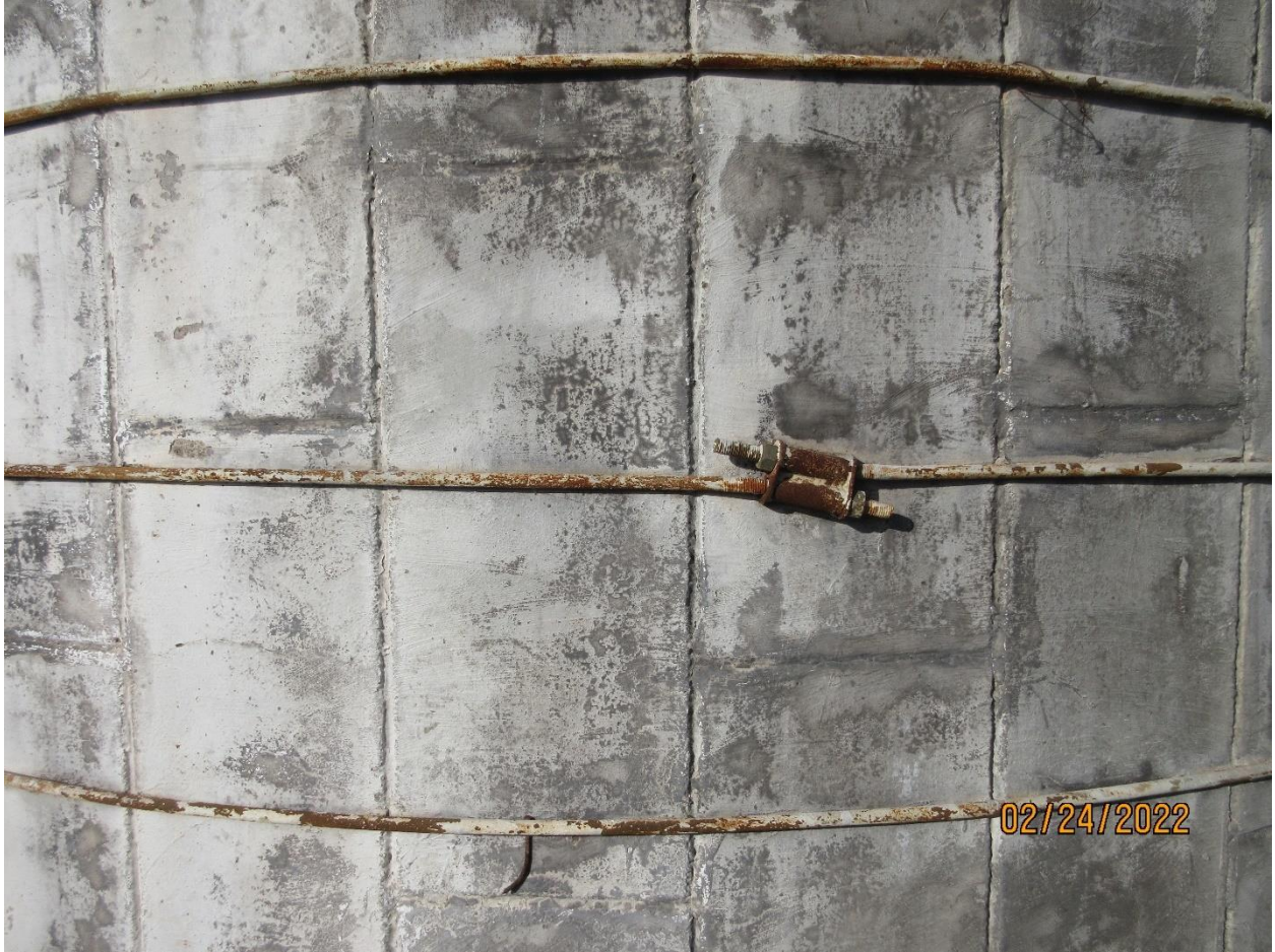
Image 16: Detail of the concrete block masonry, approximately 12" by 30", of the silos with the iron banding.
