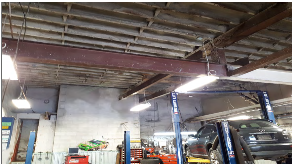
Figures 45 & 46: (above) Interior view of Florentine arched doorway within building Section 'B' (below) View of ceiling in Building Section 'B' with steel beams (Source: MHBC, 2019)
