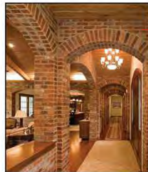
RECLAIMED BRICK ARCH
