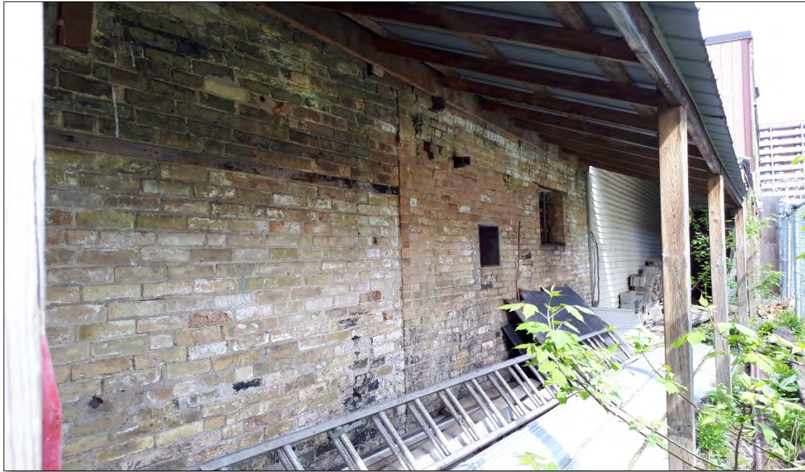
Figure 41: View of east elevation (Source: MHBC, 2019)
