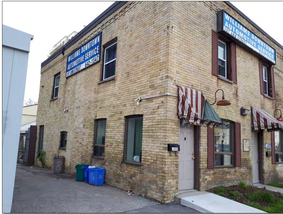
Figure 40: View of north (front) elevation (Source: MHBC, 2019)
