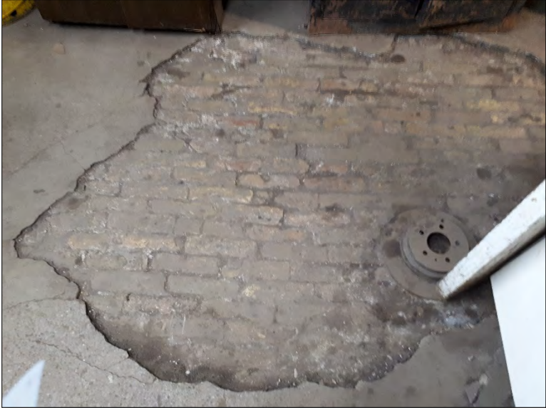
Figures 49 & 50: (above) Interior view of building Section 'C' showing corbelled brick supports in basement; (below) View of original brick flooring in basement of Section 'C' (Source:MHBC, 2019)
