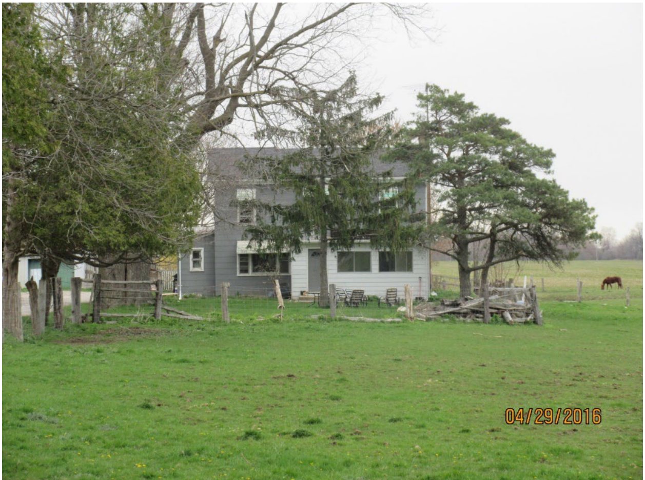
Image 2: Photograph of the farmhouse at 3700 Colonel Talbot Road on April 29, 2016.
