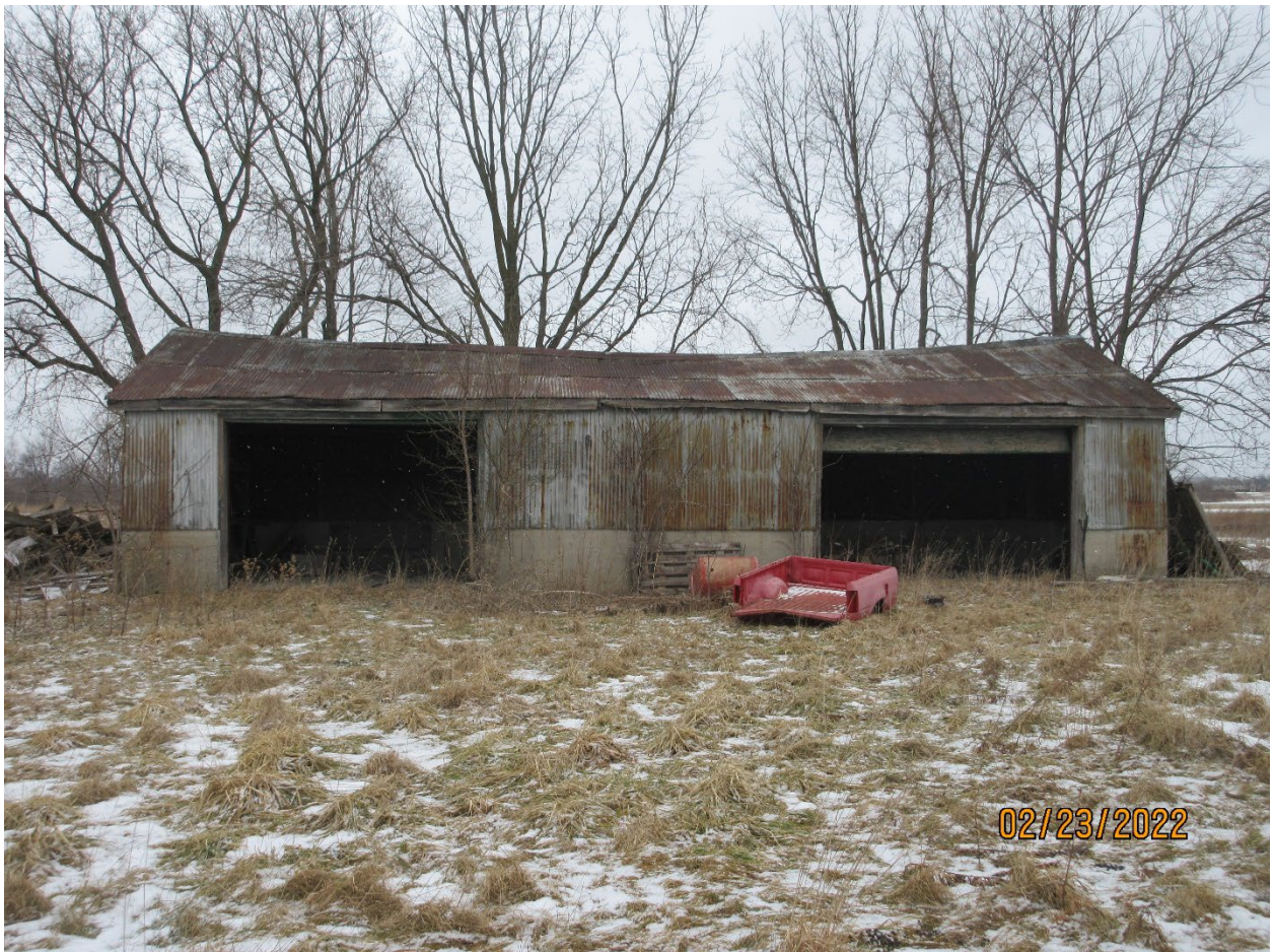
Image 12: Photograph of the driveshed at 3700 Colonel Talbot Road.
