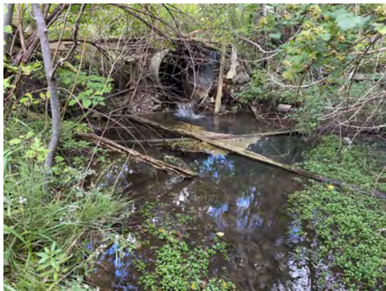
Photo 5 - September 8, 2021 Trib. C, S of Gideon Dr., looking N towards culvert outlet. Outlet is perched and discharging into pool.
