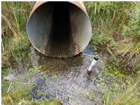
Photo 3 - September 8, 2021 Trib. C, N of Gideon Dr., looking S towards culvert inlet. Inlet is perched.
