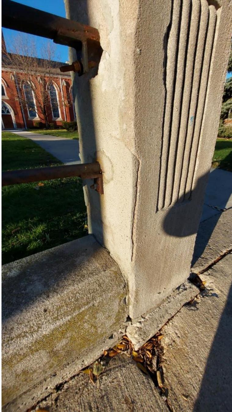
**Photograph 21:** End post with localized repairs (AECOM, November 2021)
