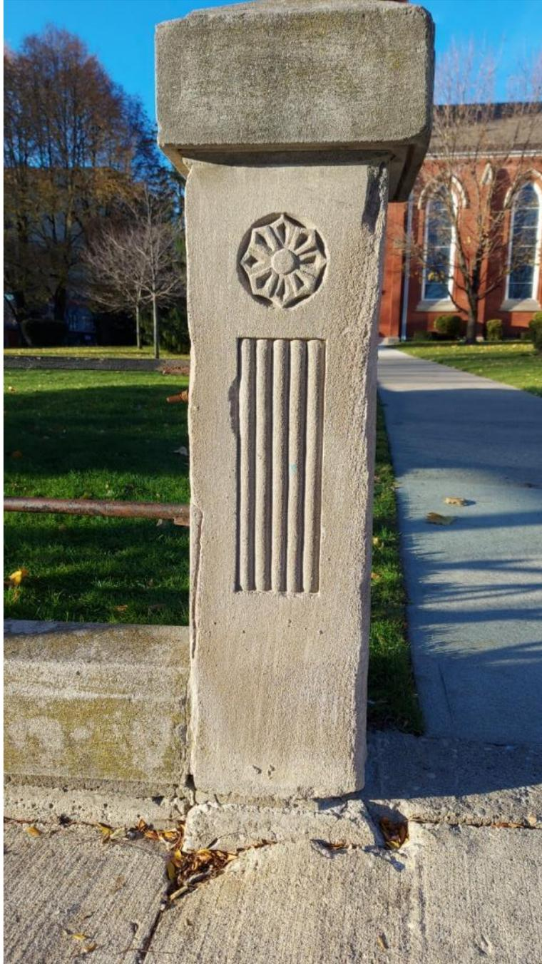
**Photograph 15:** End post proposed for relocation on Queens Avenue, showing signs of weathering and localized weathering on corners (AECOM, November 2021)
