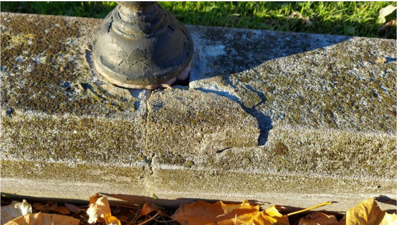
**Photograph 23:** Capstone cracking and spalling (AECOM, November 2021)
