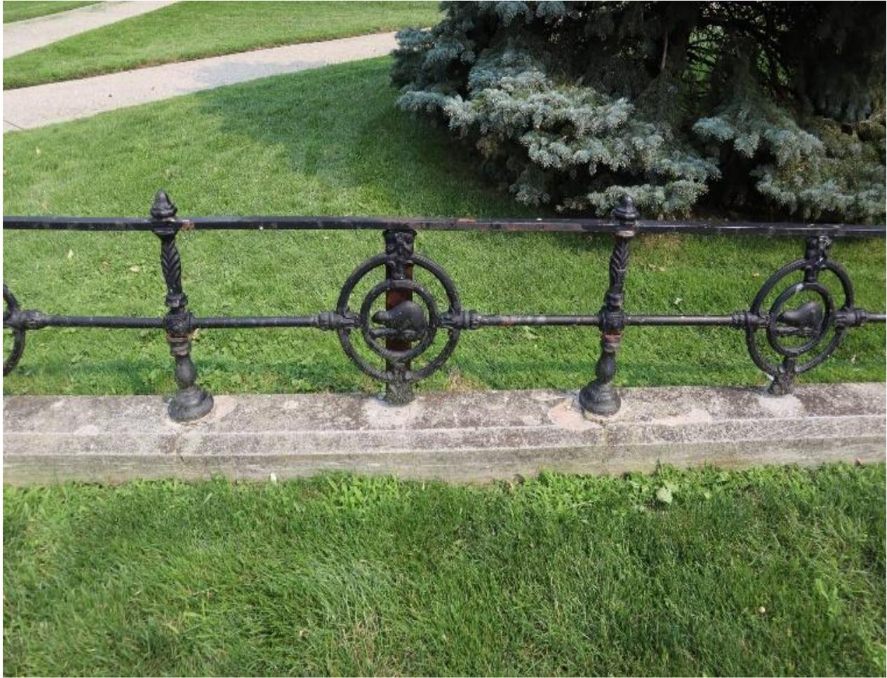
**Photograph 35:** View of the beaver fence on Queens Avenue with buried foundation (AECOM, May 2021)
