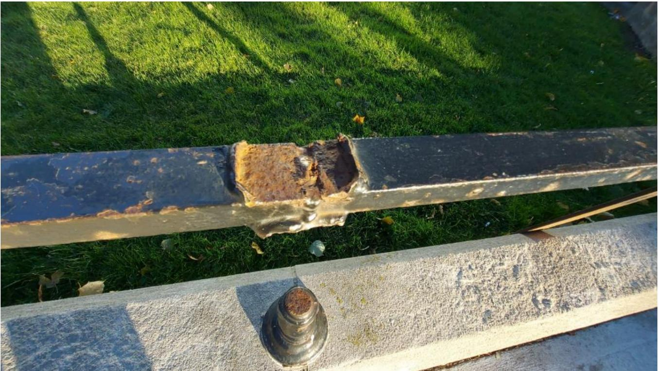
**Photograph 32:** The flat horizontal bar was placed over the vertical rail post and welded (AECOM, November 2021)
