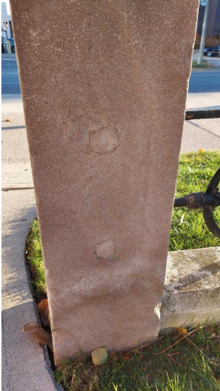
**Photograph 20:** Former holes in the end posts (for horizontal rail attachment) that were patched up, potentially indicating the end post was turned for repairs (AECOM, November 2021)
