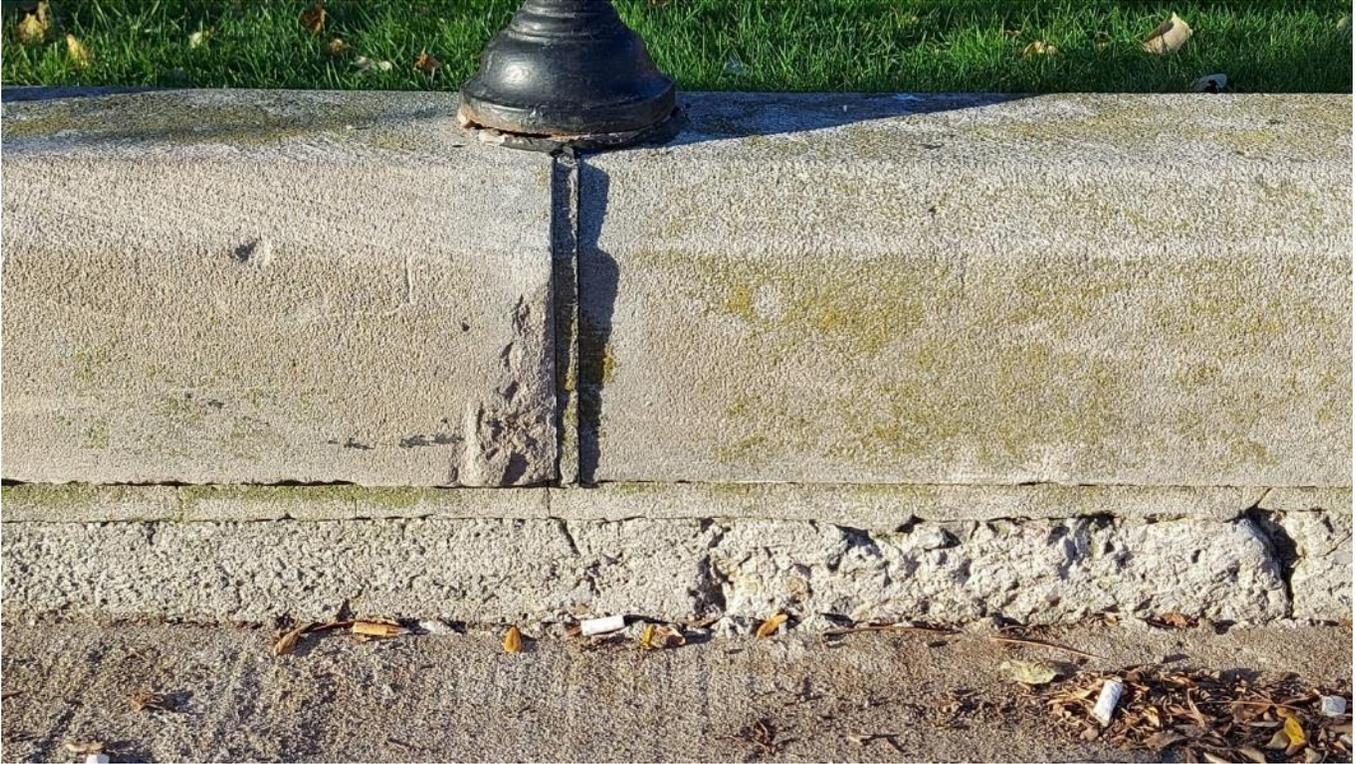
**Photograph 24:** View of mortar joint between cap stone and concrete foundation and mortar joint at each vertical rail post location (AECOM, November 2021)
