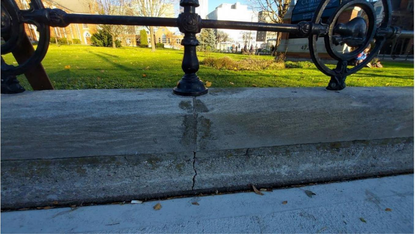
**Photograph 27:** Caulking below the base of the post to increase contact and seal area below (AECOM, November 2021)
