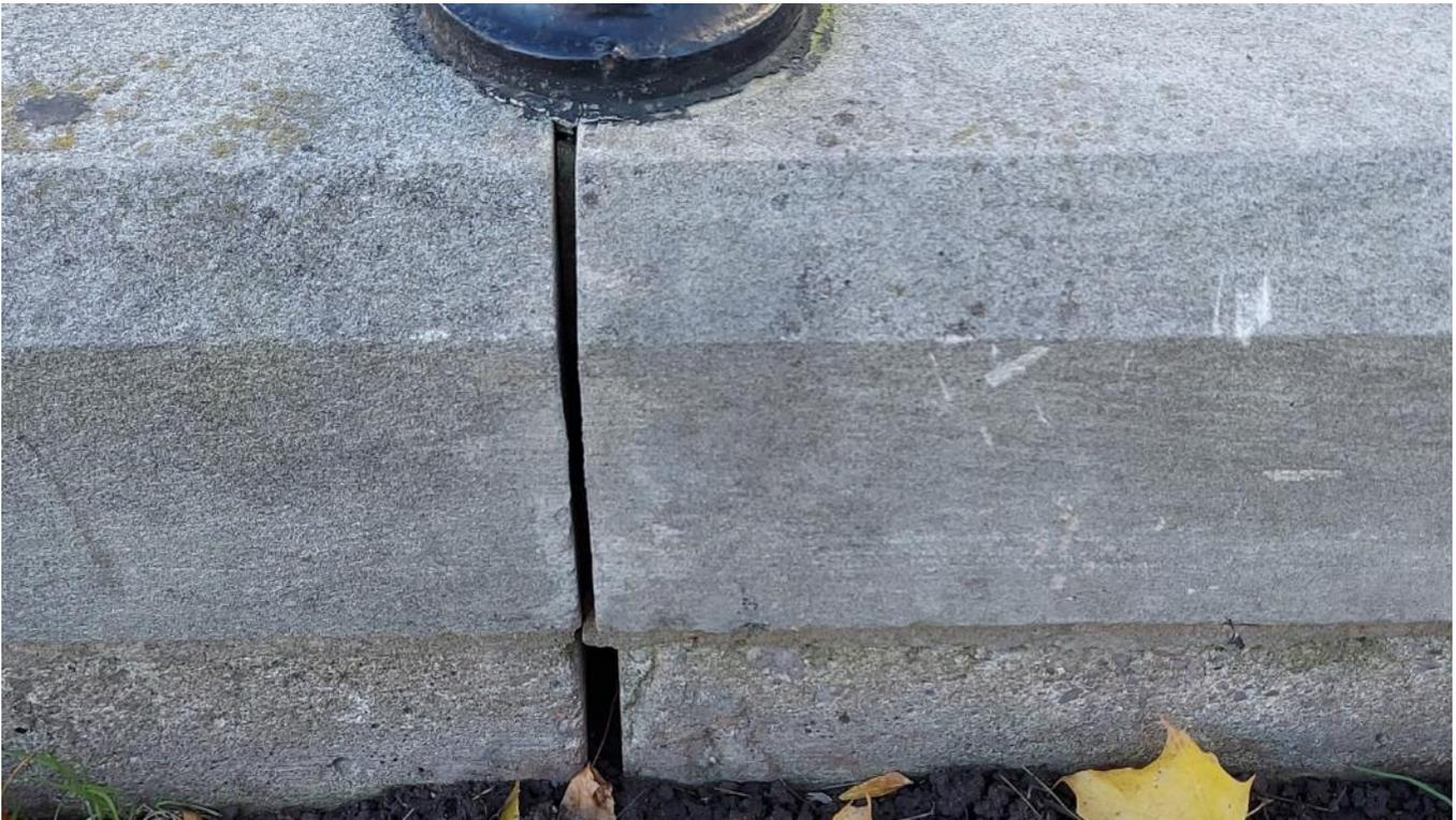
**Photograph 25:** Example of mortar joint missing and the cap stone cut and notched at each joint to accommodate the post attachment (AECOM, November 2021)
