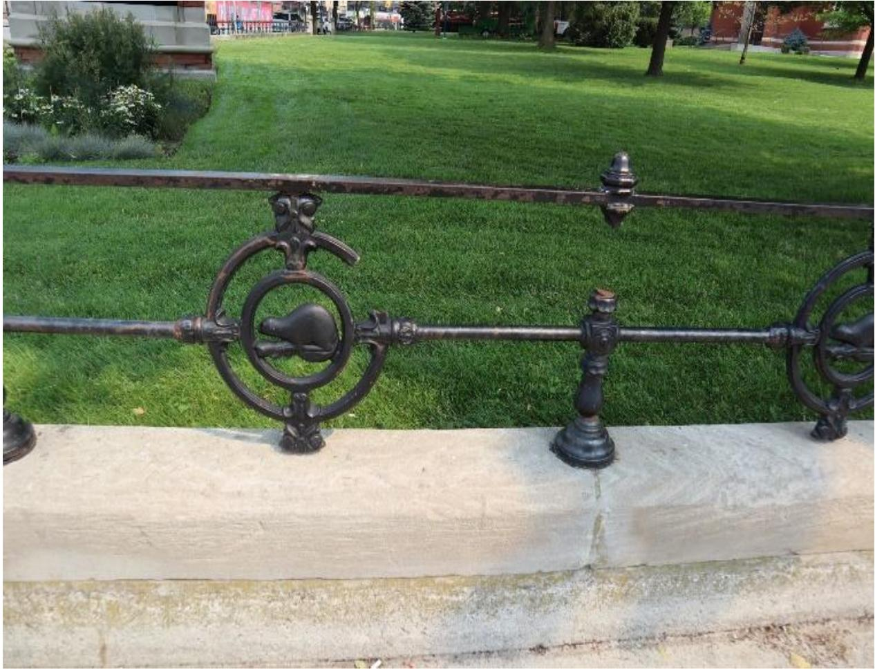
**Photograph 30:** Damaged section of the beaver fence on Richmond Street (AECOM, May 2021)
