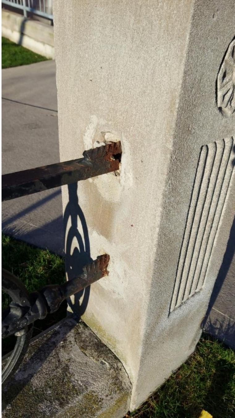
**Photograph 18:** Original arrangement with where horizontal rails mortared into end posts (AECOM, November 2021)
