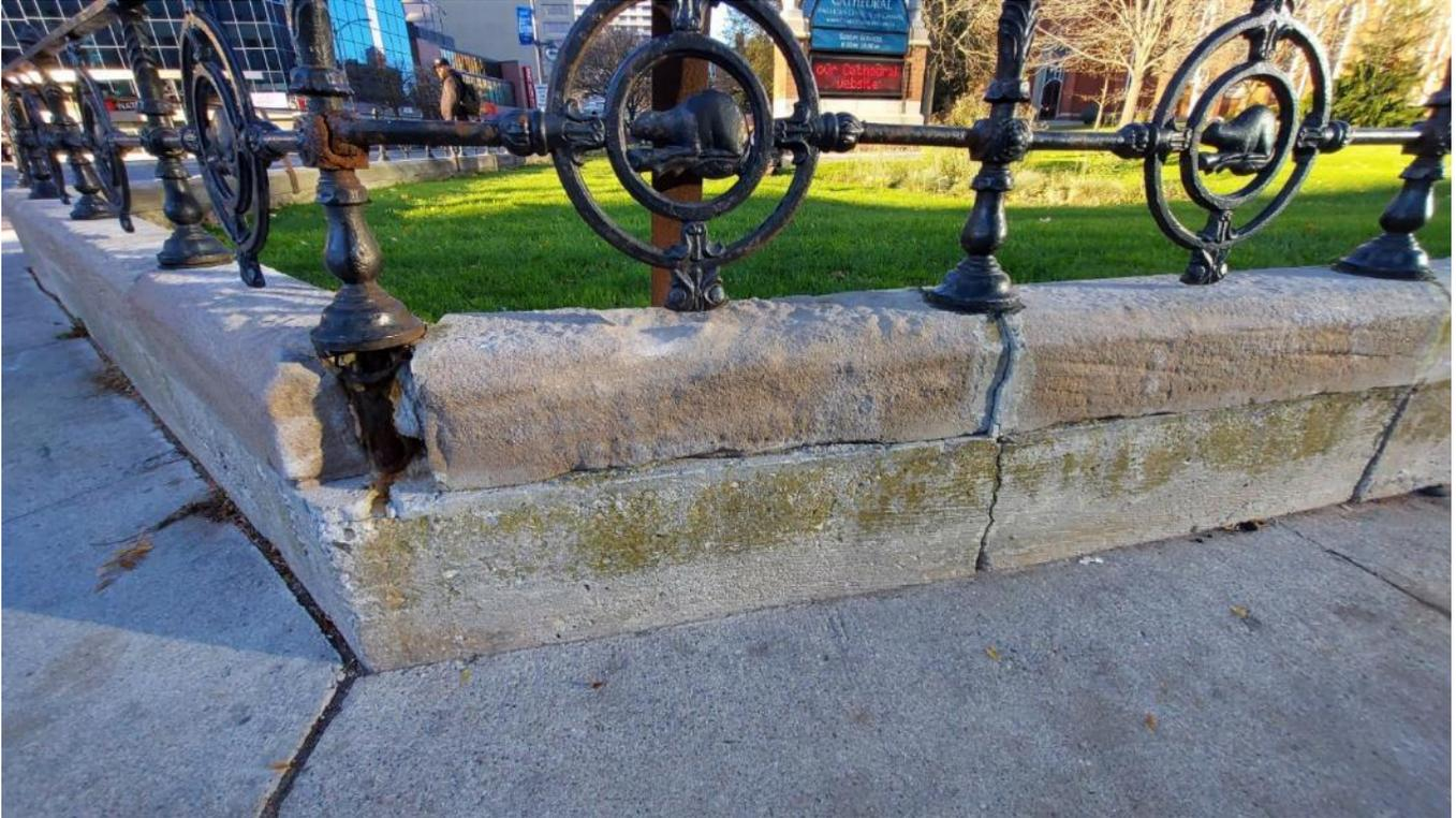
**Photograph 22:** Example of a cap stone in poor condition (AECOM, November 2021)
