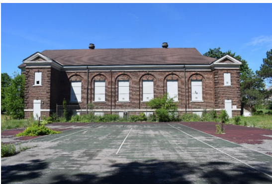
Photo 20: Recreation Hall east elevation looking west
