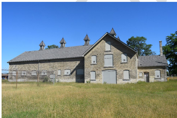
Photo 1: Horse Stable looking northwest
