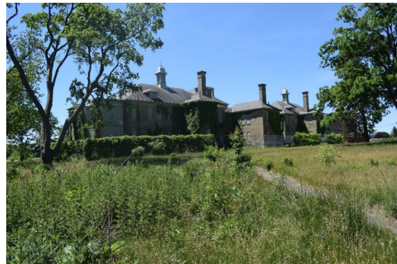
Photo 15: Infirmary north (rear) elevation looking southwest
