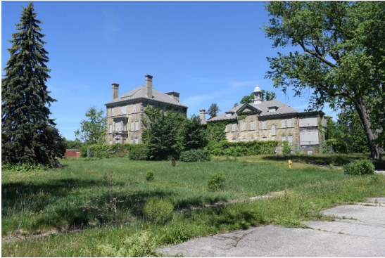
Photo 10: Infirmary south elevation looking northwest
