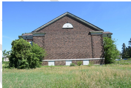
Photo 21: Recreation Hall south elevation looking north
