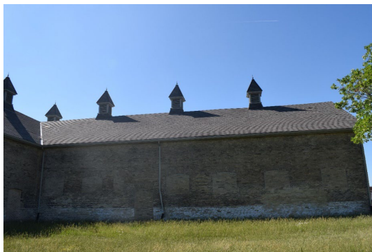
Photo 4: Horse Stable looking south
