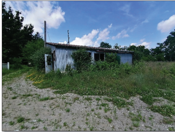
Figure 24: View of outbuilding 1 looking east (MHBC, 2021)
