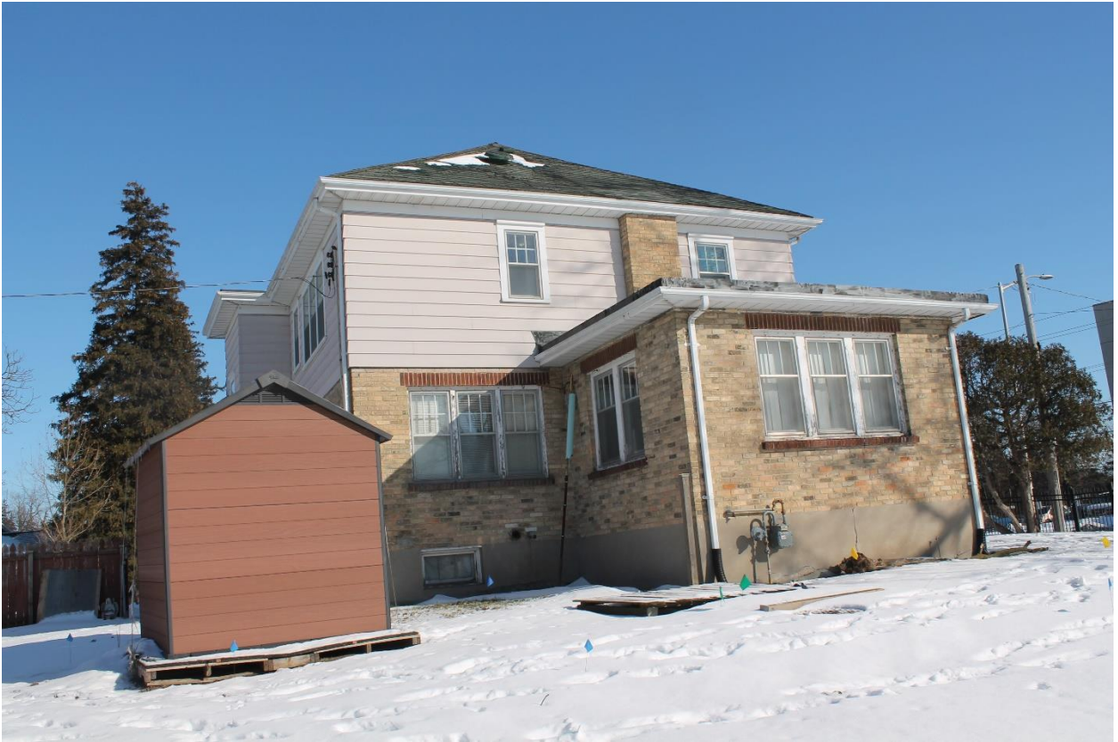
Image 7: Photograph showing the west (rear) elevation of the former gate house (2022).
