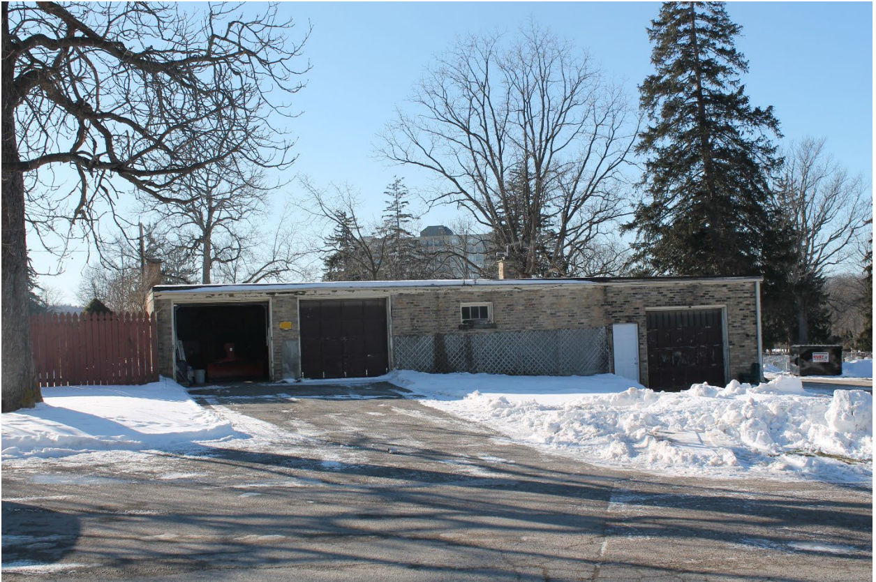
Image 9: Photograph showing the front elevation of the maintenance garage (2022).
