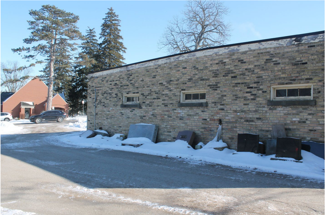
Image 10: Photograph showing the side elevation of the maintenance garage and the new administrative office at left (2022).
