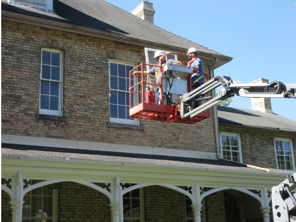
Image 2: Work underway to install the recently restored storm windows at Grosvenor Lodge.
