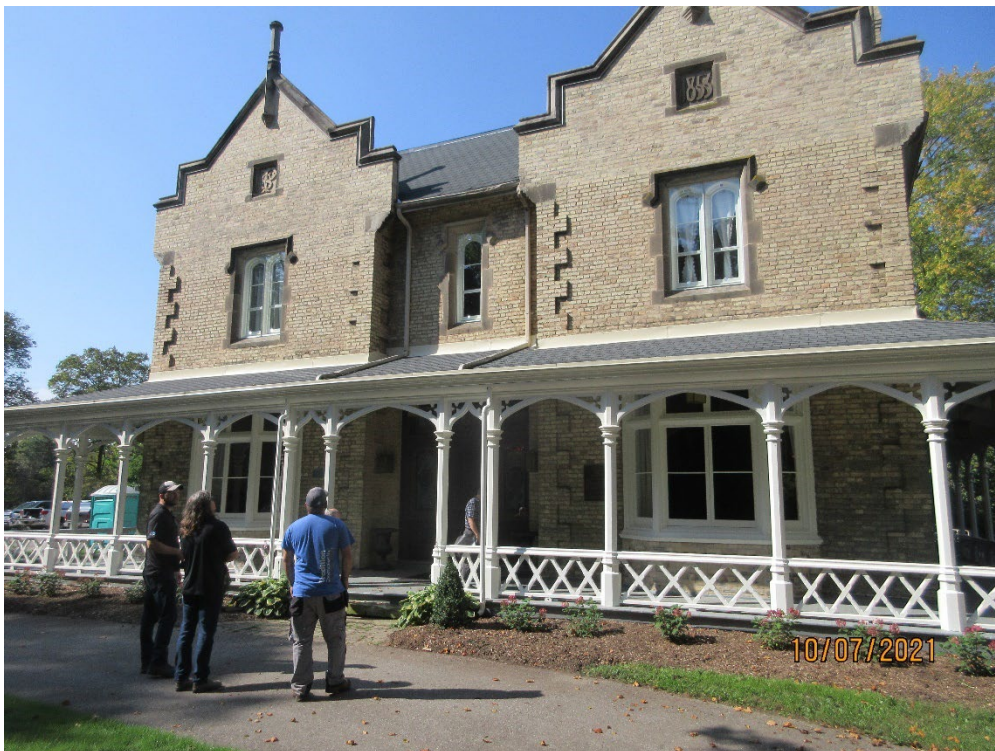
Image 3: Inspecting the new "Cathedral style" storm windows on the upper front windows at Grosvenor Lodge.
