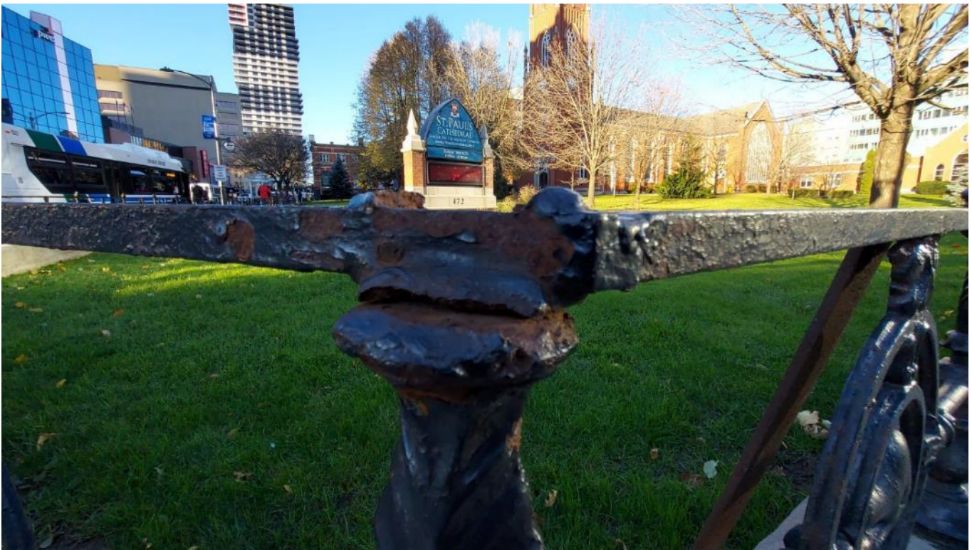
Photograph 34: Welding with cracks, illustrating piece by piece on-site construction of fence (AECOM, November 2021)
