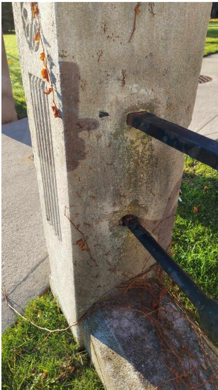
Photograph 19: Modified horizontal rails which place reinforcing steel bars into holes with mortar and welding of reinforcing steel bars to horizontal rails (AECOM, November 2021)
