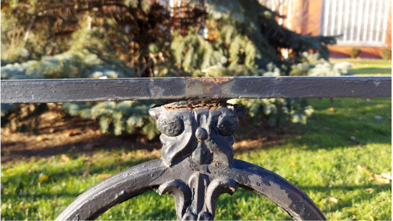
Photograph 33: Beaver medallion welded to top horizontal rail (AECOM, November 2021)
