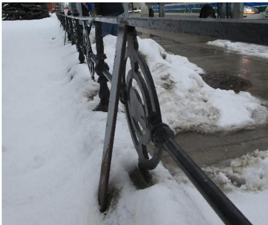
Photograph 40: Example of the back-support brace (AECOM, February 2021)
