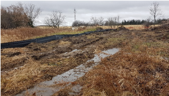
Photo 5. Pooled water within future Bradley Avenue road allowance. View towards southwest.
