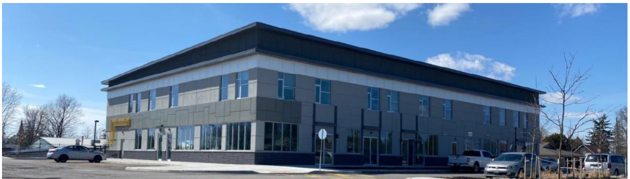
Figure 3: Office to the north
