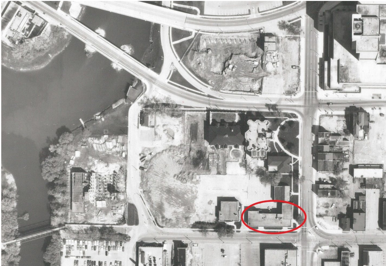
Image 8: Aerial photograph from 1978 annotated to show the building at 50 King Street (circled in red). The old Police Station has been demolished, and demolition is underway on the Penman's Factory (now Ivey Park) as well as the Exchange Building (now the lawn of Museum London at 421 Ridout Street North). The City Registry Office, the County Registry Office, and the County Building (Surrogate Court Building) are still extant at the time of the photograph in 1978.
