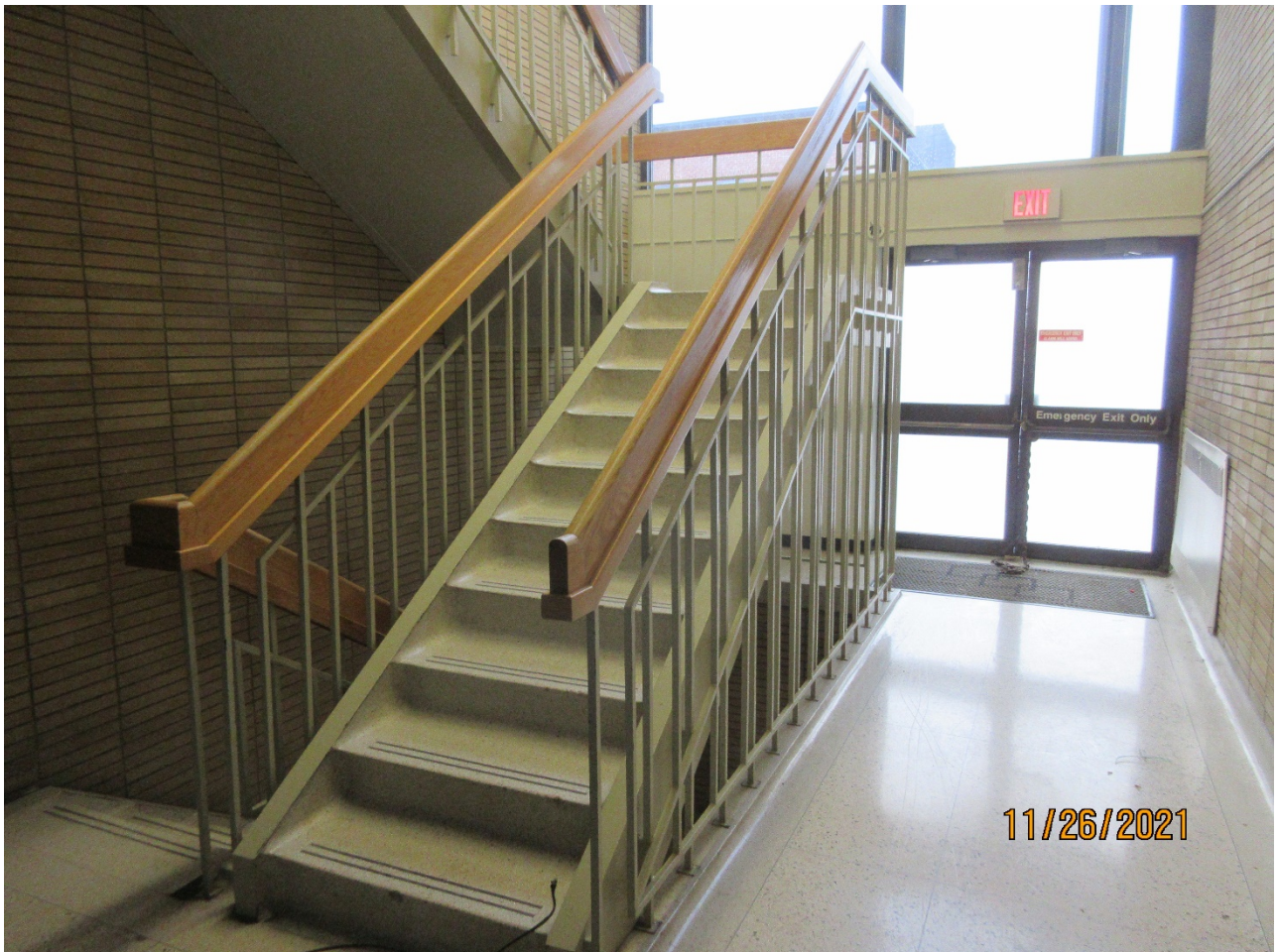
Image 15: This photograph, showing the westerly staircase/stairwell with the doors onto King Street, shows some of the few remnants of the 1959 building's details: terrazzo flooring, stacked roman bricks, and the staircase.
