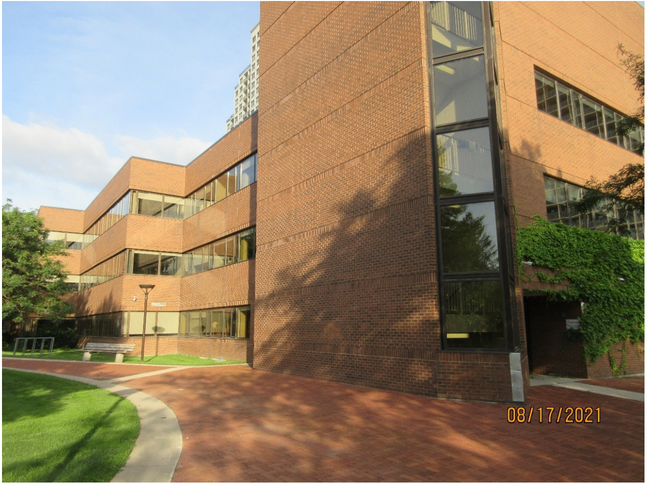
Image 14: Detail of the west and north elevations of the building on the property at 50 King Street.
