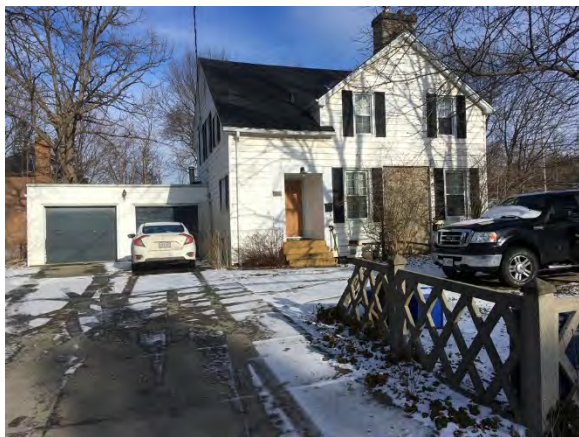
Plate 7: Front (south) façade of 368 Windermere Road, looking north (concrete fence is also visible)
