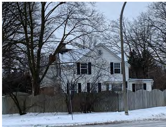
Plate 8: East façade of 368 Windermere Road, looking west
