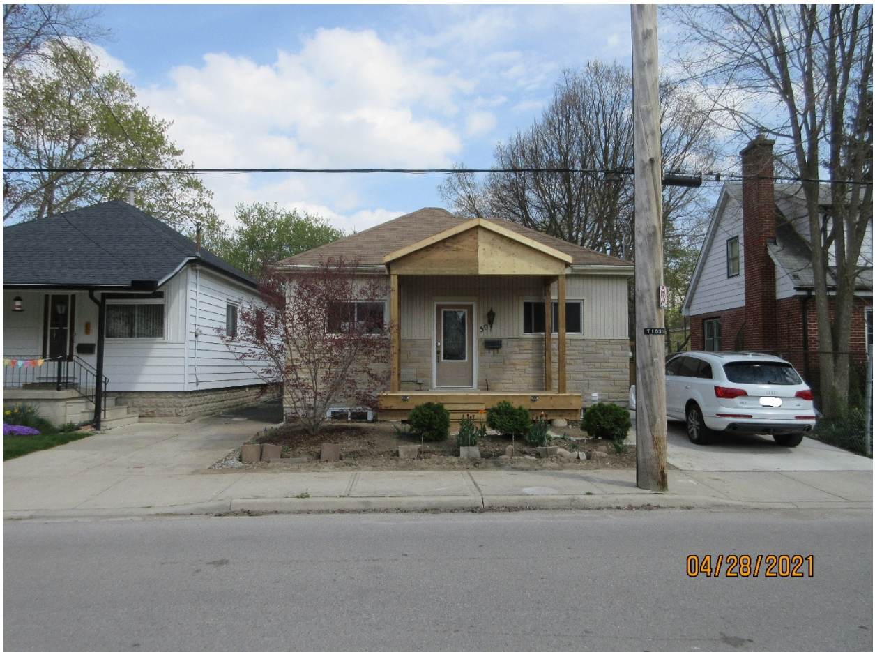
Image 2: Photograph of the dwelling located at 59 Albion Street showing the porch under construction in spring of 2021.
