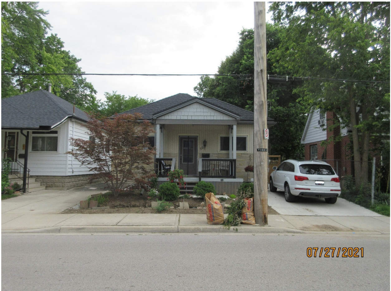
Image 4: Photograph of the dwelling located at 59 Albion Street, as observed in July 2021 showing unapproved railing system.
