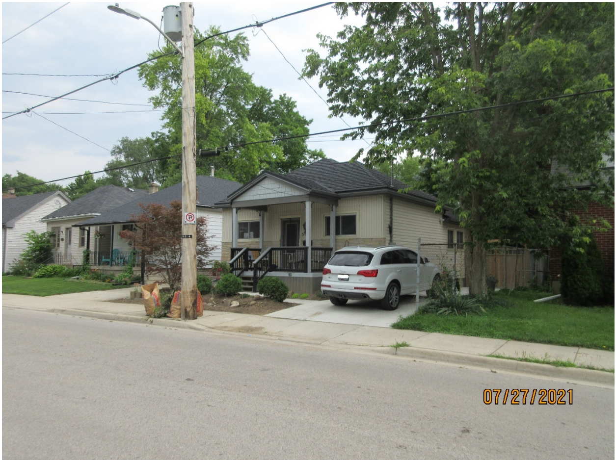
Image 3: Photograph of the dwelling located at 59 Albion Street, as observed in July 2021 showing unapproved railing system.
