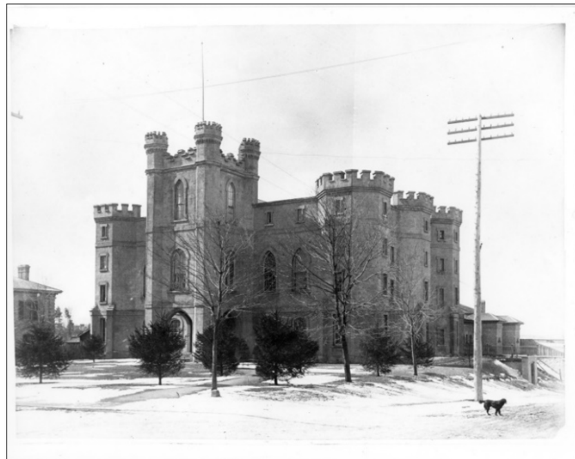
Figures 26 & 27: (above) Photograph of the courthouse and landscaping in 1933 (Source: Seale Family); (below) Photograph of the Middlesex County Courthouse 1939 with the County Office in the background to the left of the photograph (Courtesy of Western University Library).
