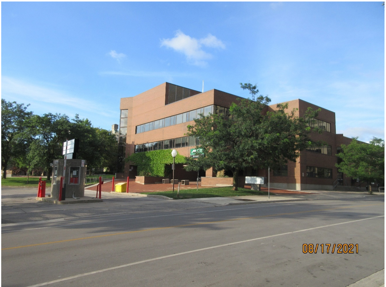
Image 13: South (King Street) and west elevations of the building on the subject property at 50 King Street. The main entrance is located under the umbrage (overhang).
