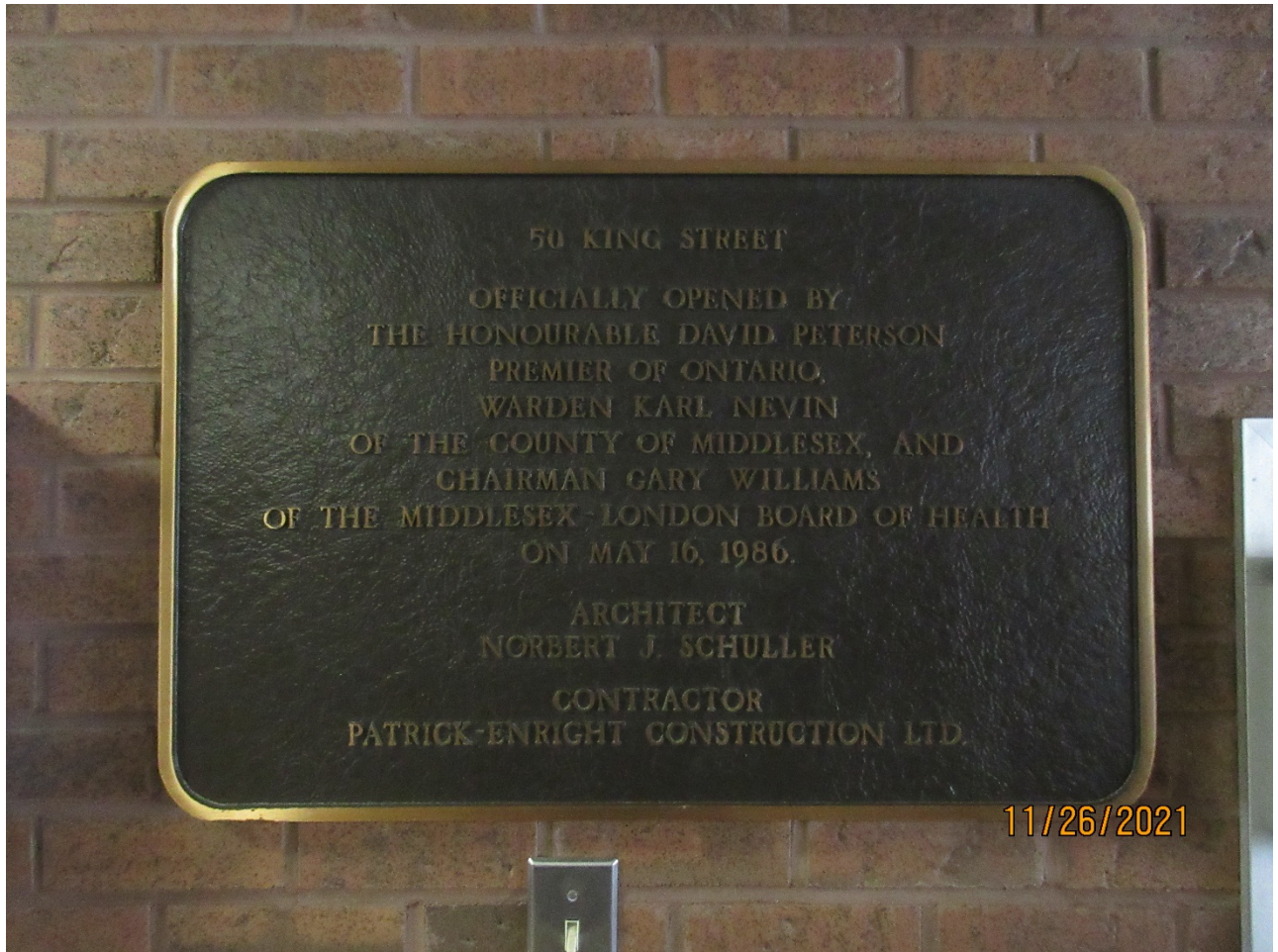
Image 18: Plaque commemorating the opening of the building at 50 King Street by Premier David Peterson on May 16, 1986, installed in the main (west) vestibule.
