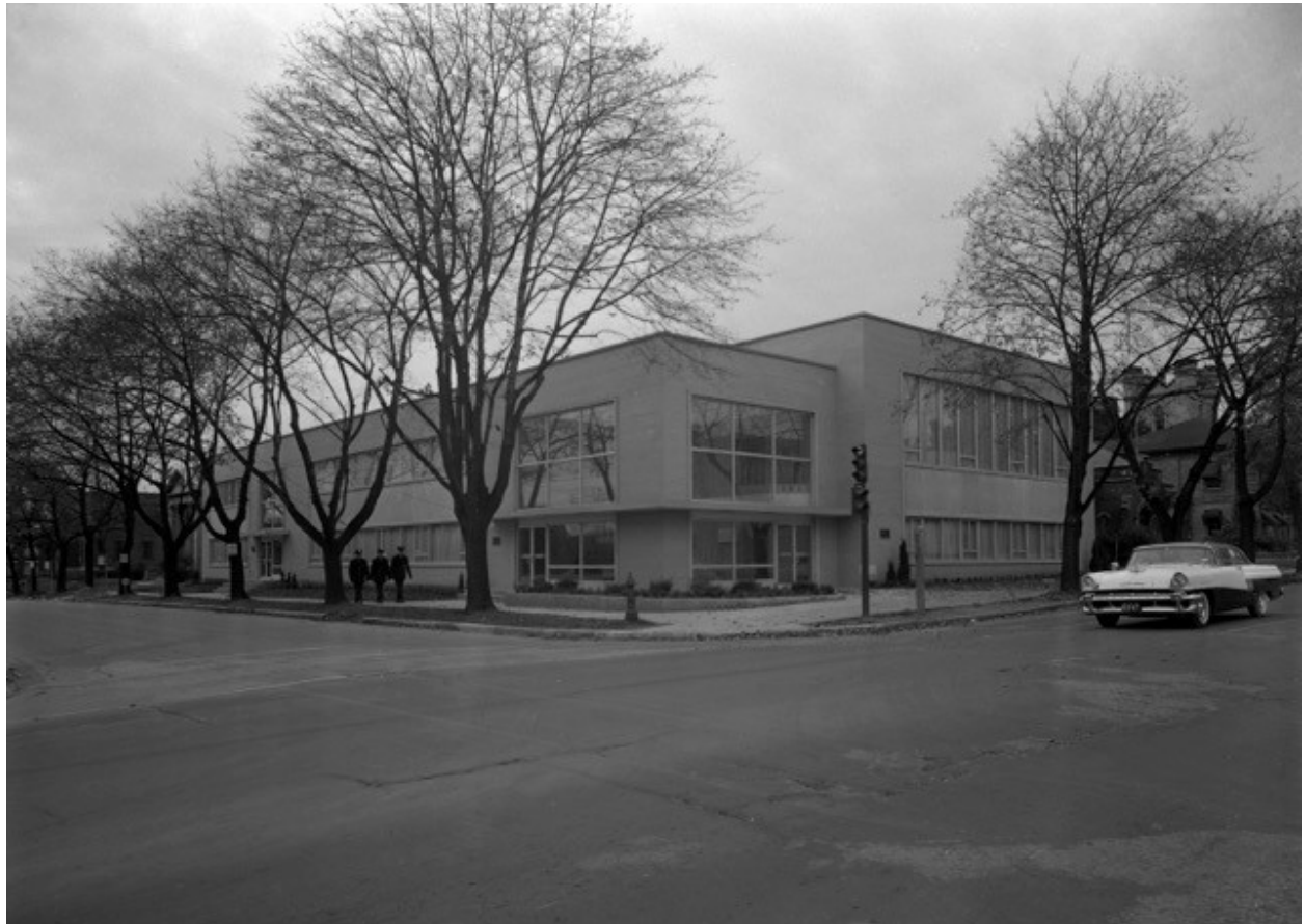
Image 6: View of the south and east façades of the Middlesex Municipal Building taken shortly after its construction in 1959. Courtesy Archives and Special Collections, Western University.
