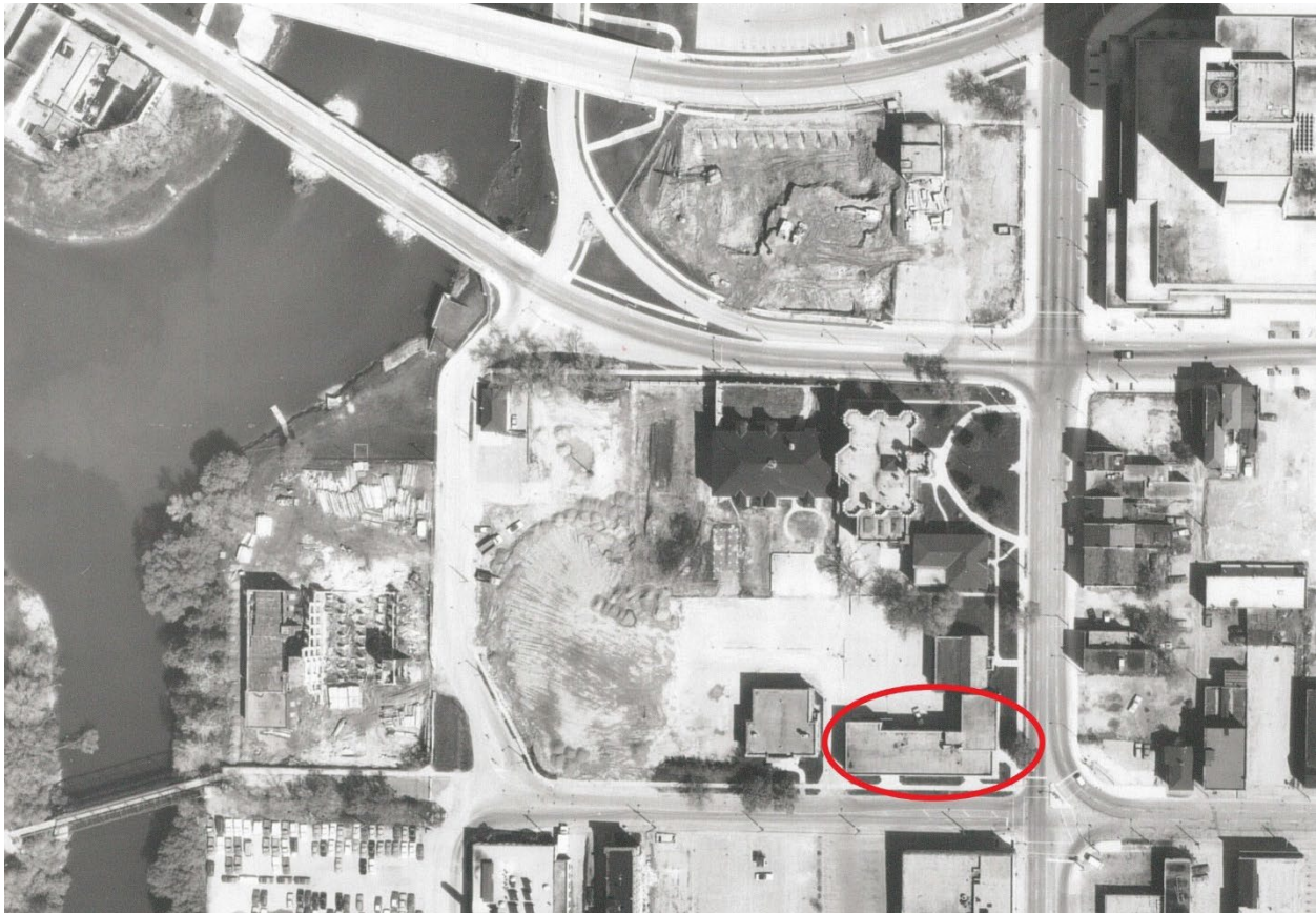
Image 8: Aerial photograph from 1978 annotated to show the building at 50 King Street (circled in red). The old Police Station has been demolished, and demolition is underway on the Penman's Factory (now Ivey Park) as well as the Exchange Building (now the lawn of Museum London at 421 Ridout Street North). The City Registry Office, the County Registry Office, and the County Building (Surrogate Court Building) are still extant at the time of the photograph in 1978.
