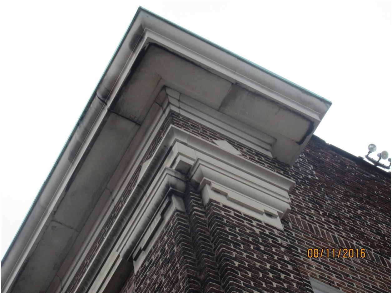
Image 6: Detail showing pilasters and cornice on the Health Services Building.
