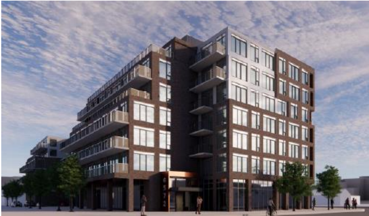
Figure 5: View along Dundalk Drive looking southeast
