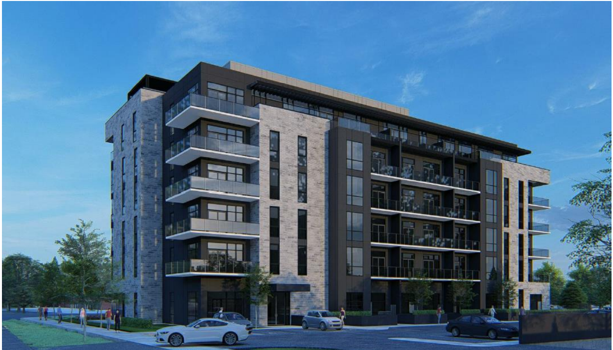
Figure 9: Revised View looking toward Southwest from Dearness Drive
