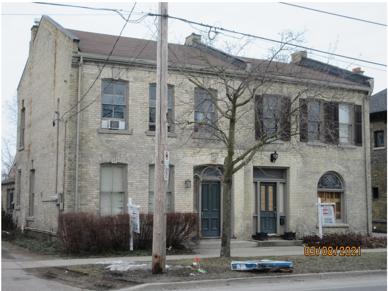
Image 3: Photograph showing the subject properties at 466-468 Queens Avenue, March 2021.
