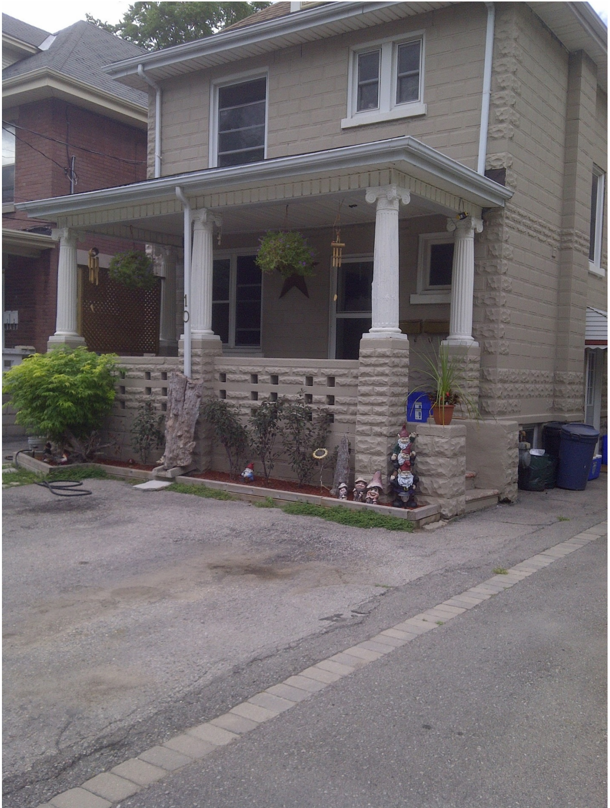
Image 2: Photograph submitted with the Heritage Alteration Permit application showing the previous appearance of the porch. The proposed alterations are to reconstruct the porch to replicate its previous design.
