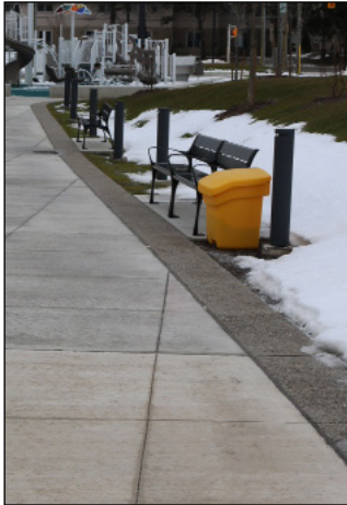
Example of the use of high colour / tonal contrast to define edge of exterior accessible route, City of London.
