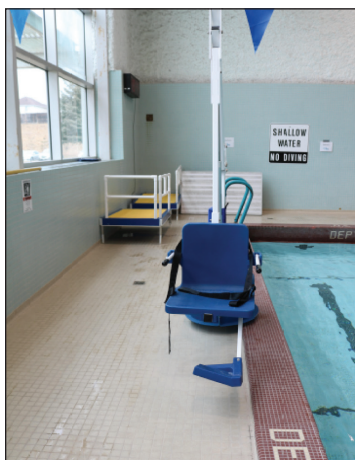
Example of pool transfer lift, City of London.
