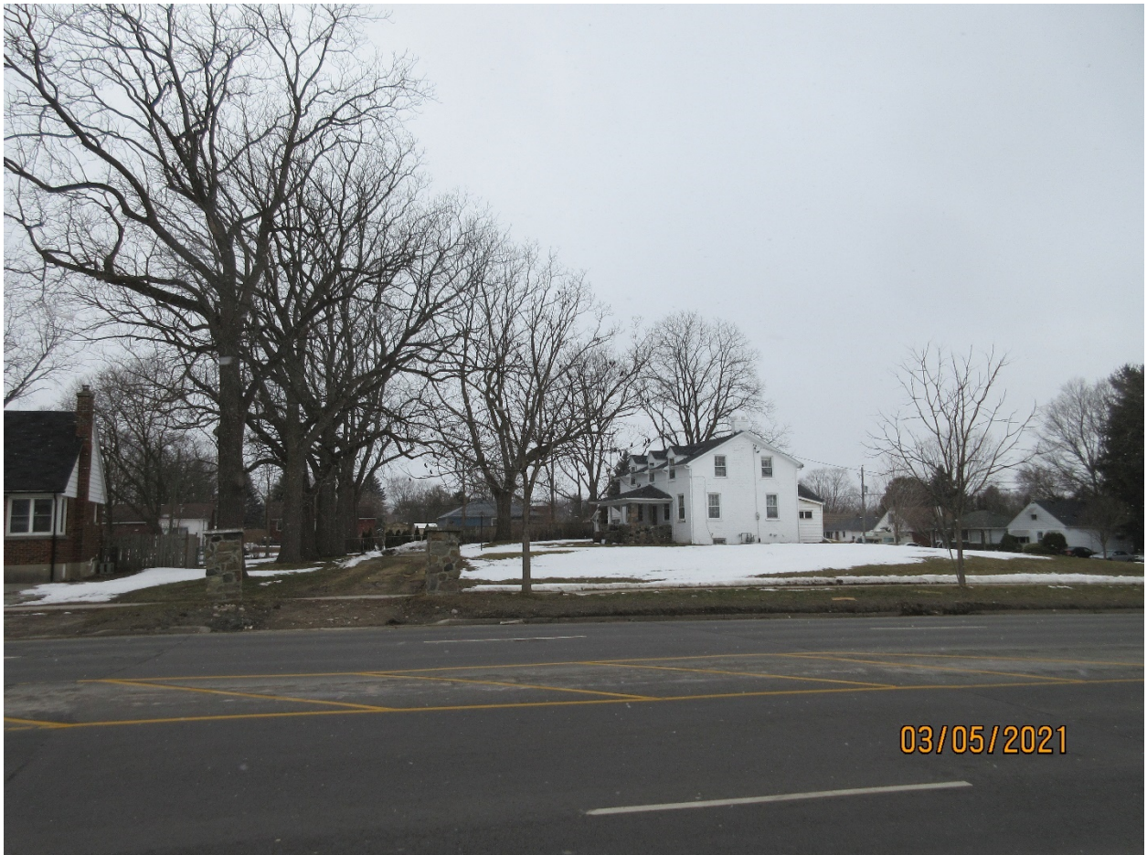
Image 2: Clarke House, as seen from the east side of Clarke Road.
