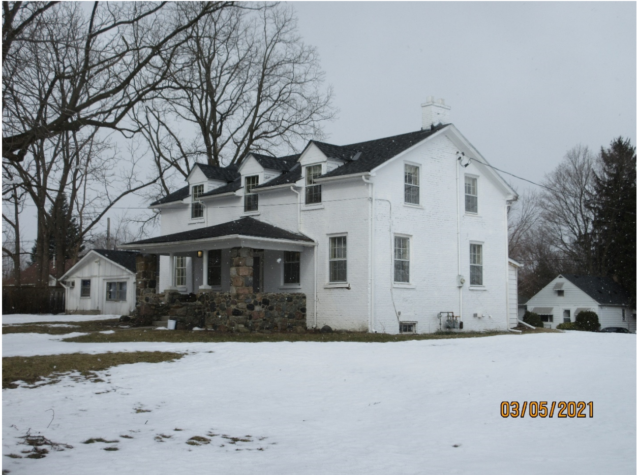
Image 5: View of the Clarke House, looking northeast from the gate posts at Clarke Road.
