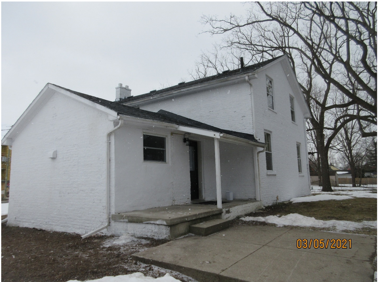
Image 10: View showing the north and west elevations of the Clarke House.
