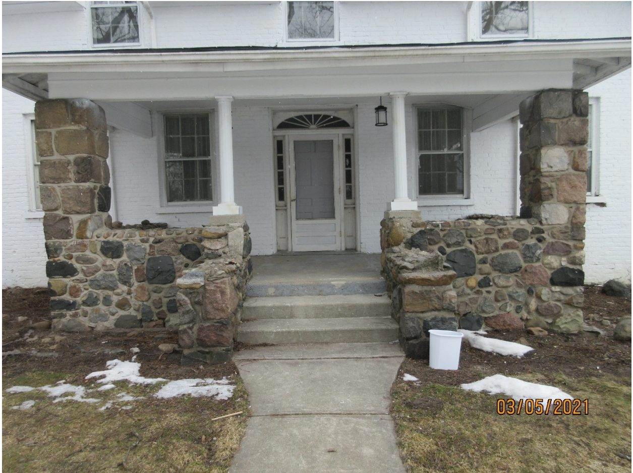
Image 13: Detail of the porch on the main (south) elevation of the Clarke House.
