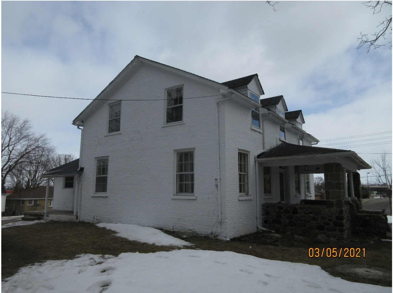
Image 11: View showing the west and south elevation of the Clarke House.
