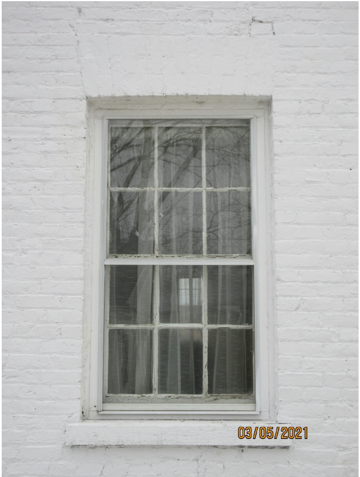
Image 17: Representative image of the six-over-six wood windows on the ground storey and gable ends of the Clarke House. The dormer windows closely resemble these windows.
