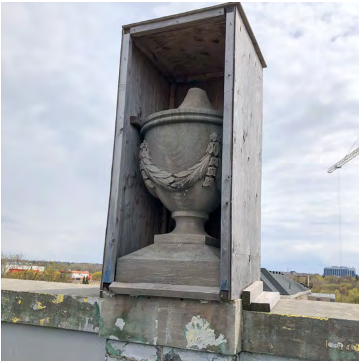
MAIN ELEVATION – classical urn on the roof
