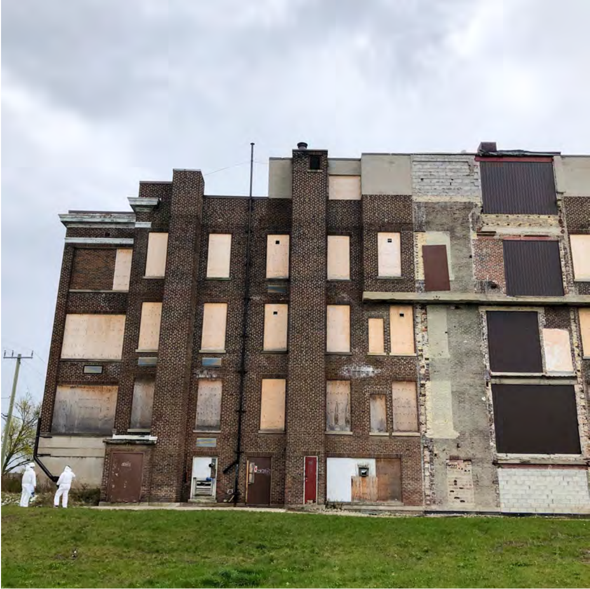
REAR ELEVATION – rear additions have been demolished
