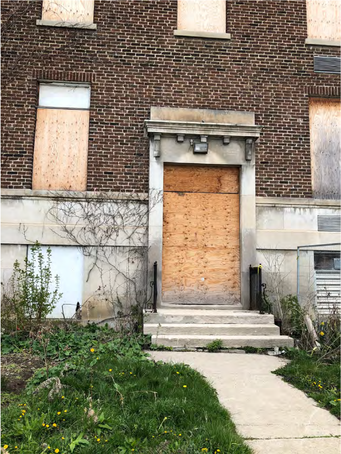
MAIN ELEVATION – SECONDARY ENTRANCE
