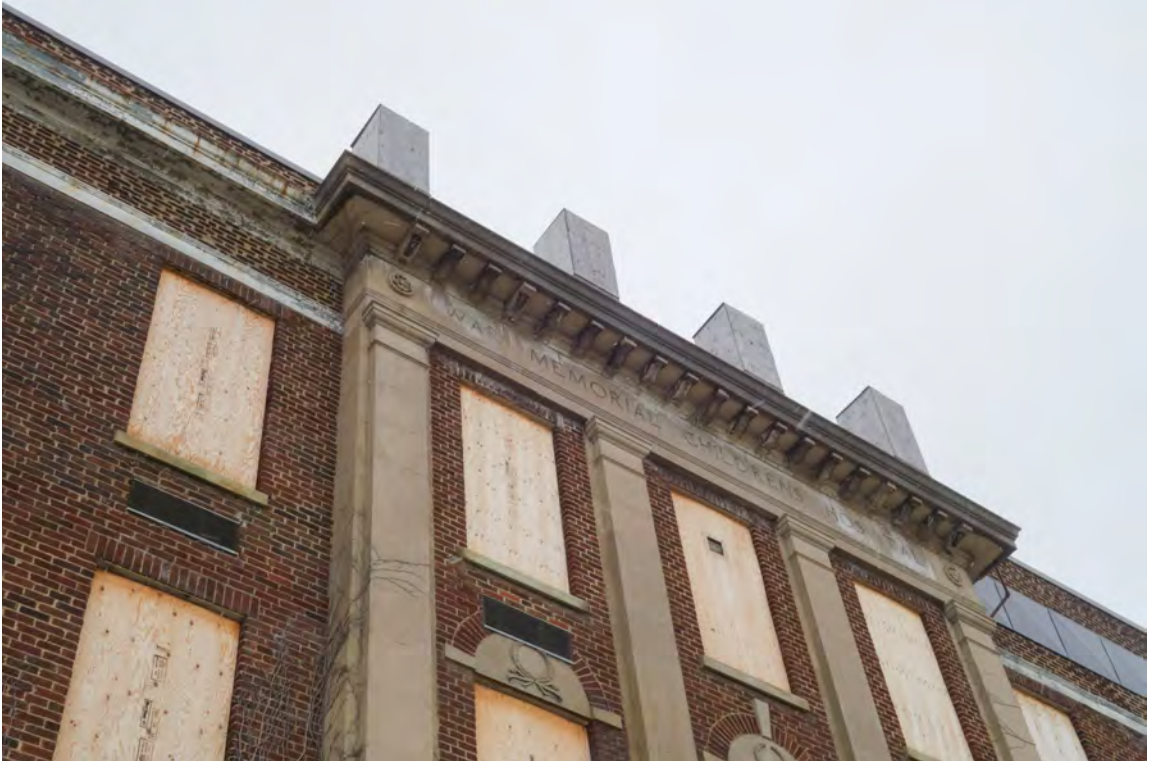
MAIN ELEVATION – four urns on the roofline with protective plywood covering
