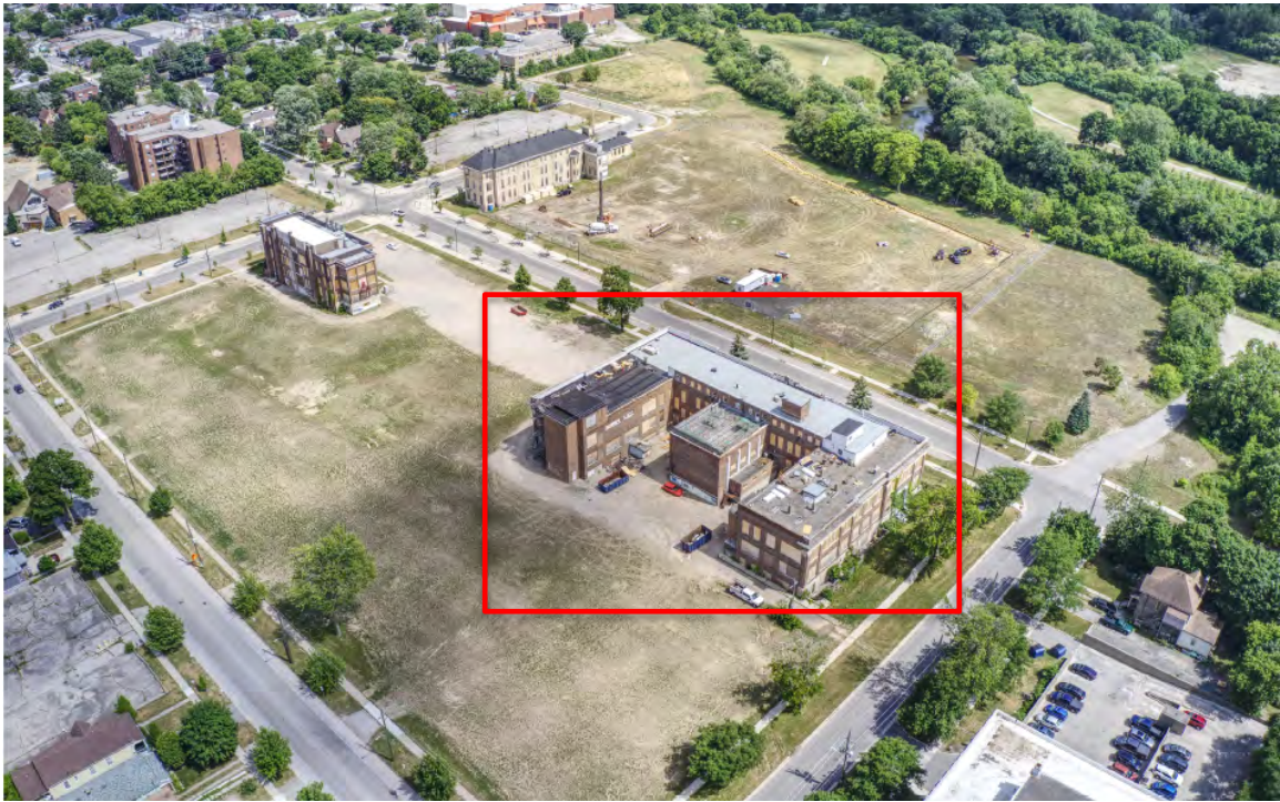
AERIAL VIEW – REAR ELEVATION
