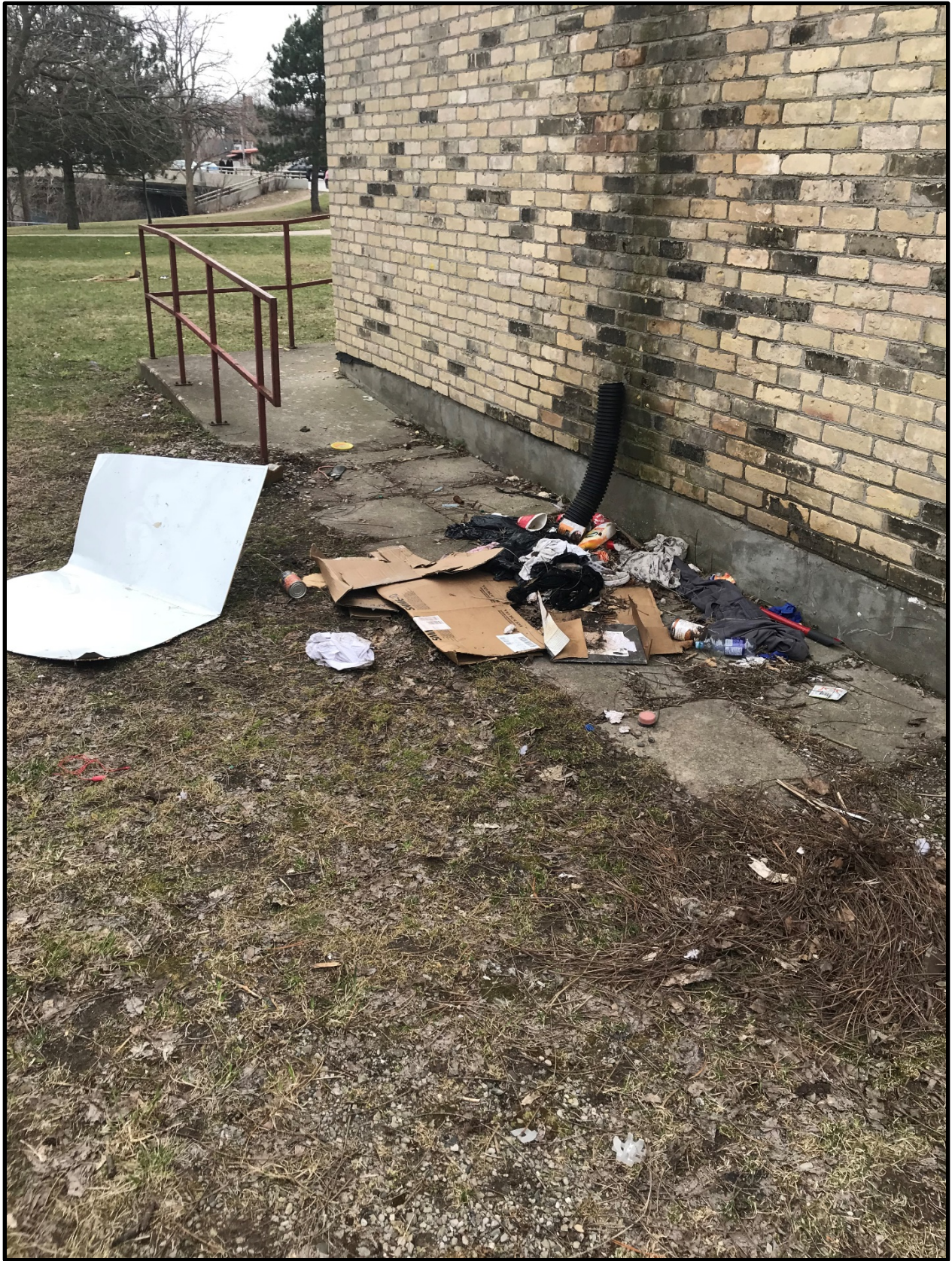
Photo 3 - rear of 72 Wellington St.
