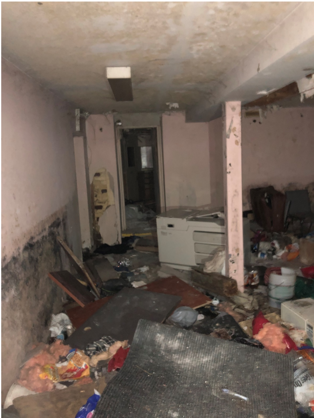
Photo 2 – Interior of 72 Wellington St.
