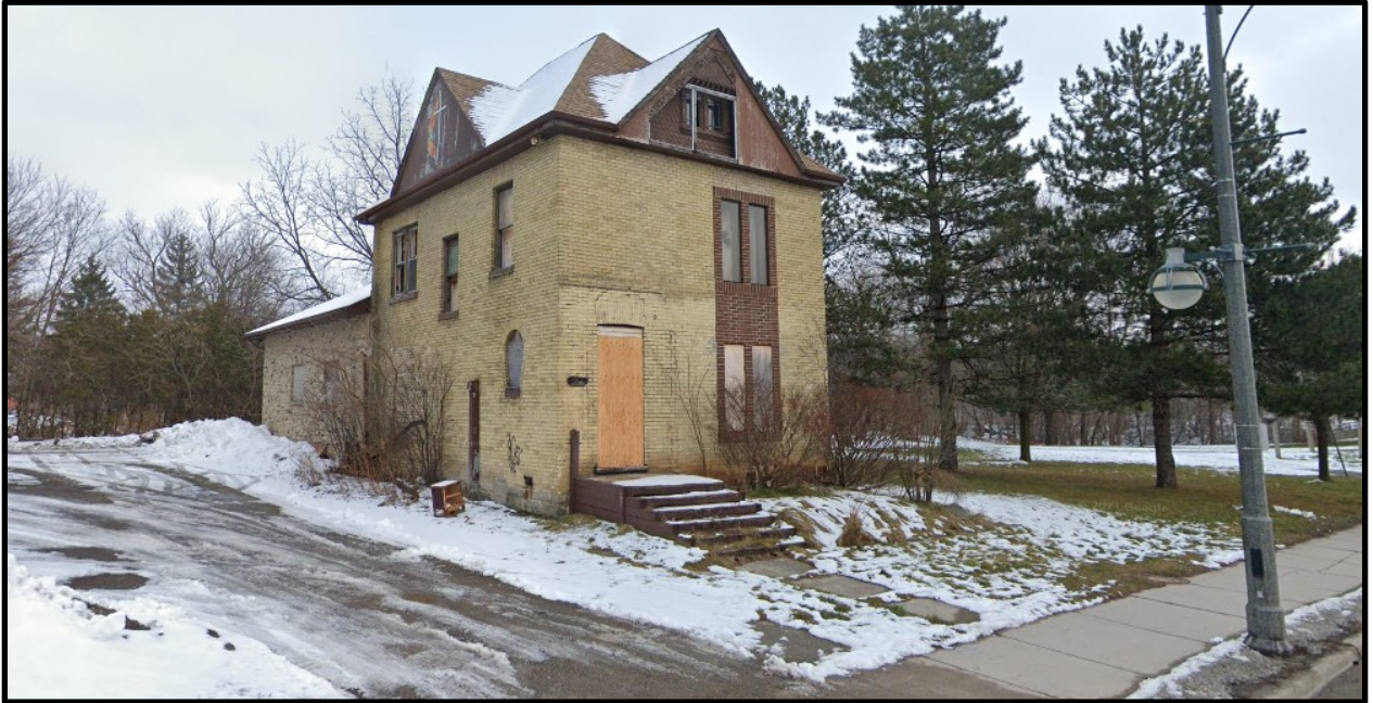
Photo 1 – 72 Wellington St. from Road
