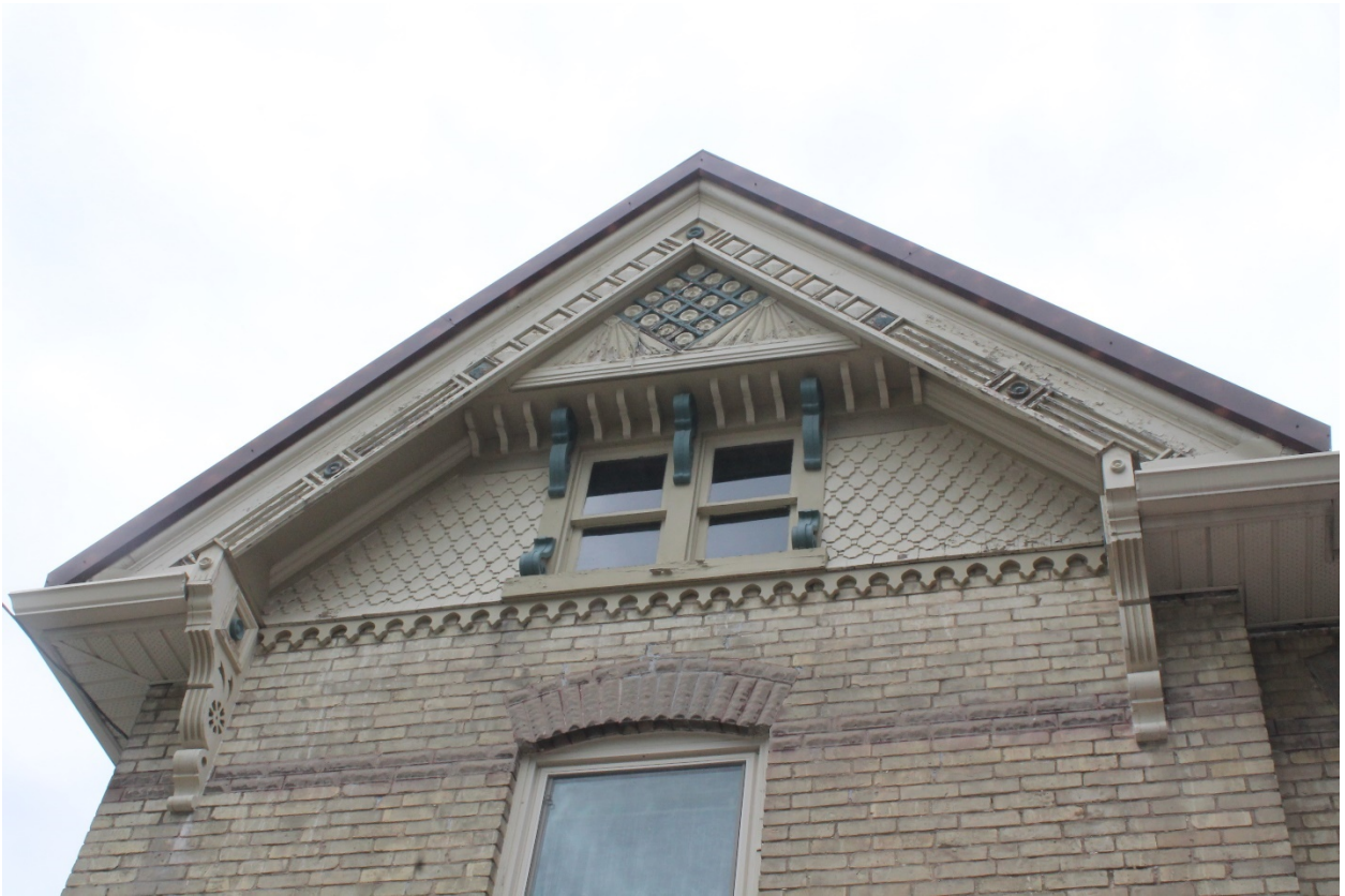
Image 6: Photograph showing the projecting gable on the front facade with decorative wood detailing.
