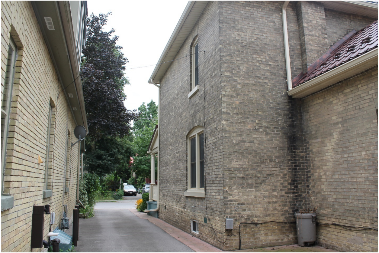
Image 3: Photograph looking south, showing the east facade of the dwelling (at right). Note the dwelling on the left is the adjacent property at 46 Bruce Street.
