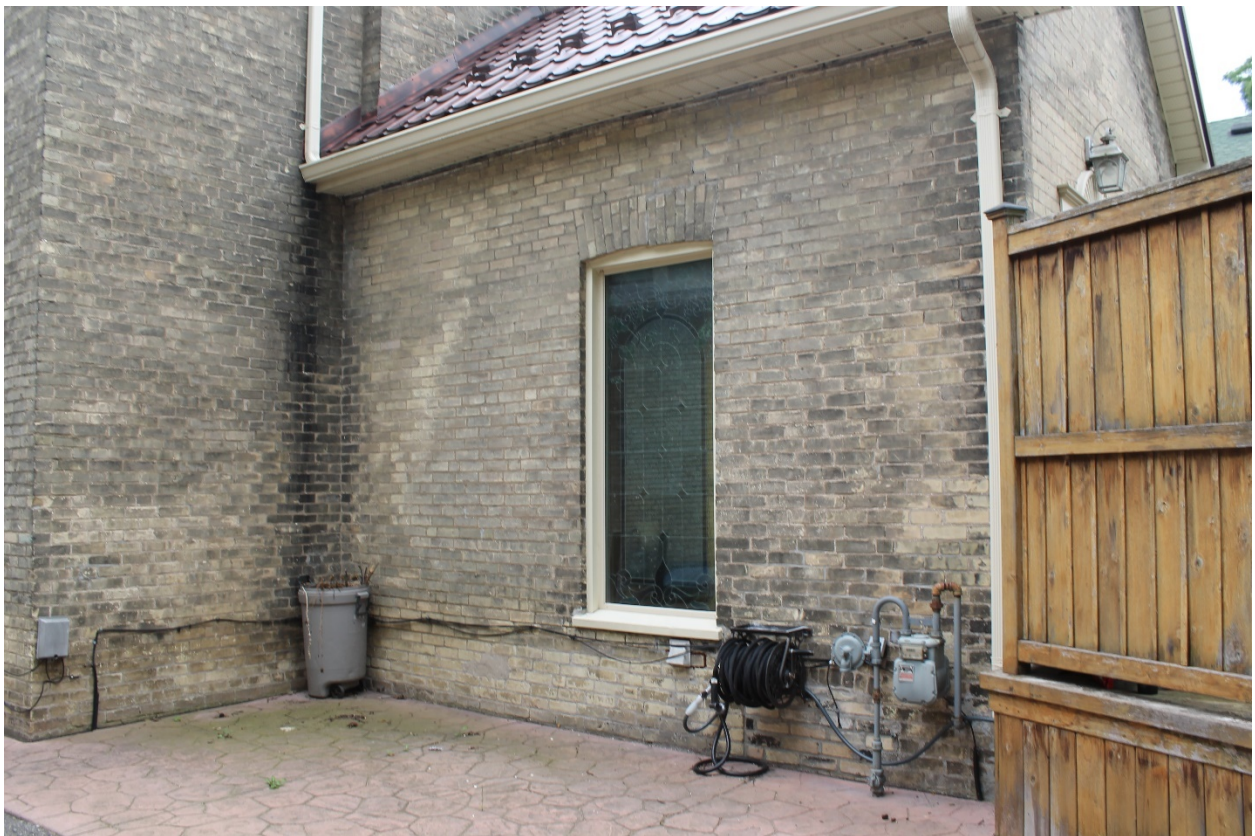
Image 4: Photograph showing the east elevation of the rear addition with casement window and stained-glass.
