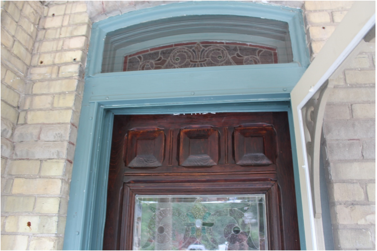
Image 11: Photograph showing door detail and stained-glass transom window.
