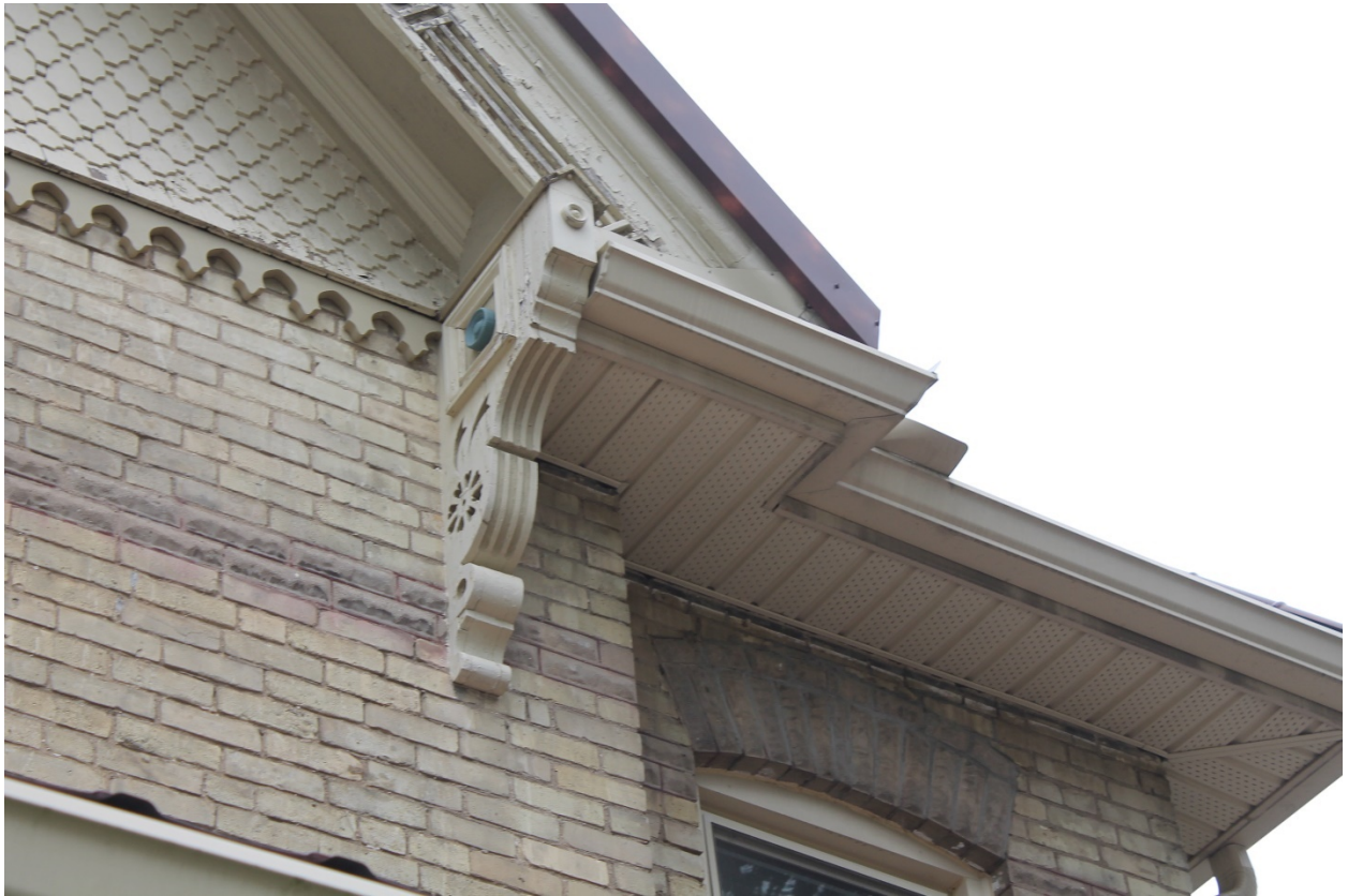
Image 10: Photograph showing details in gable and decorative brackets.
