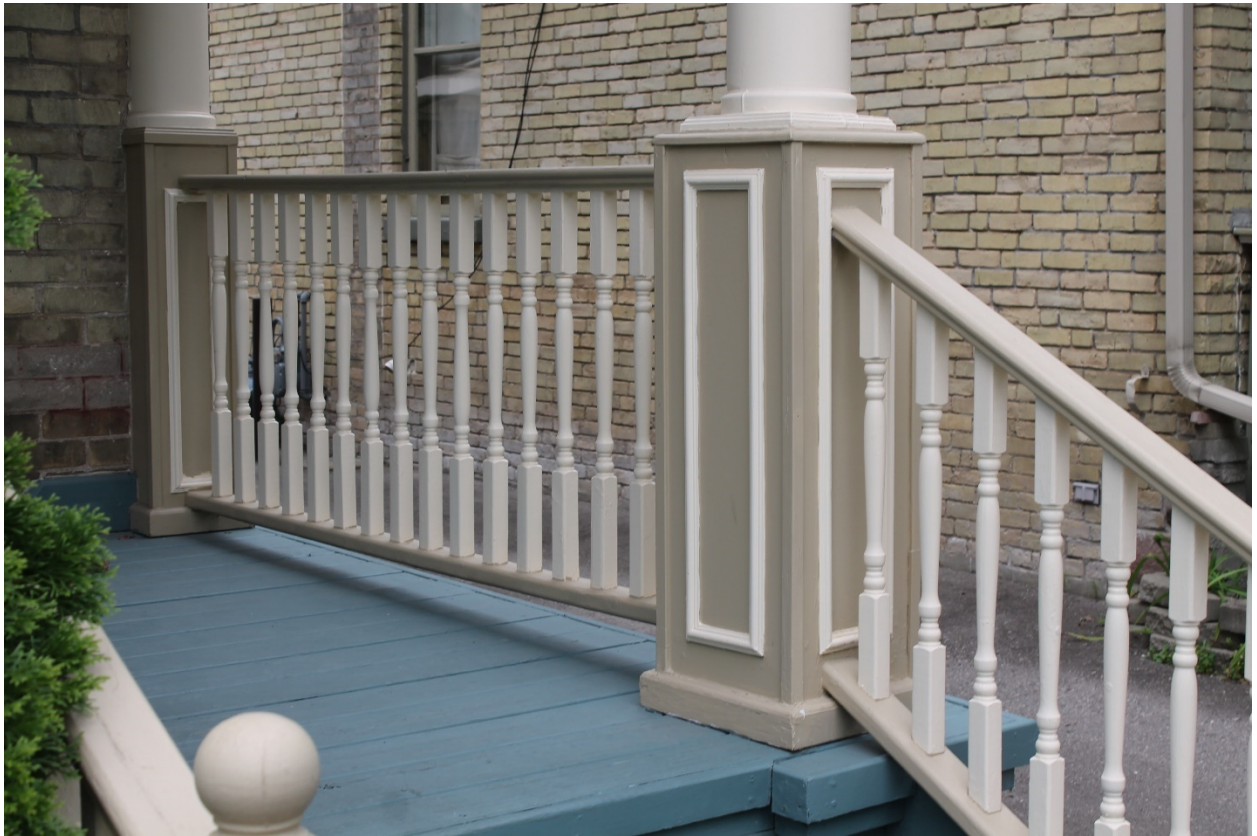
Image 14: Photograph showing details of porch columns and railing system.
