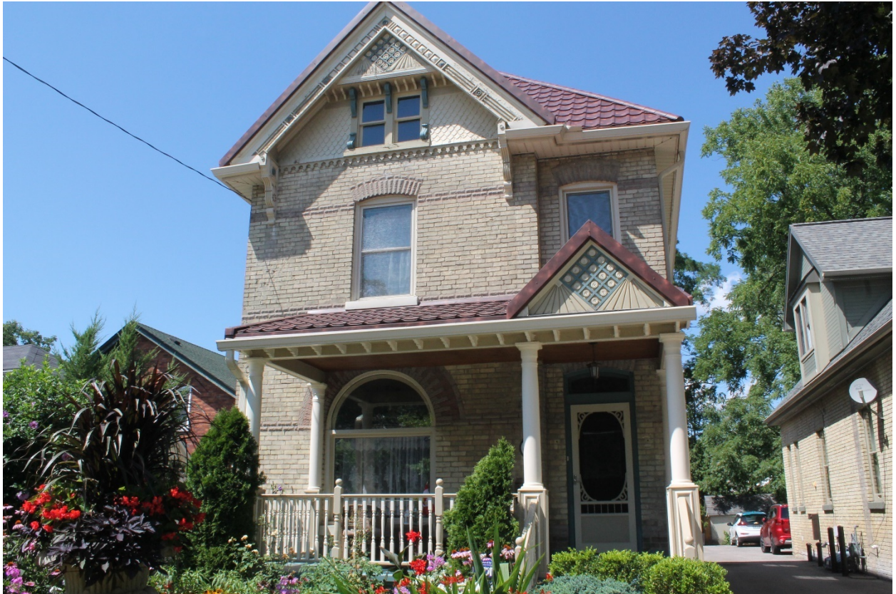
Image 1: Photograph of the south (front) facade of the dwelling at 44 Bruce Street.
