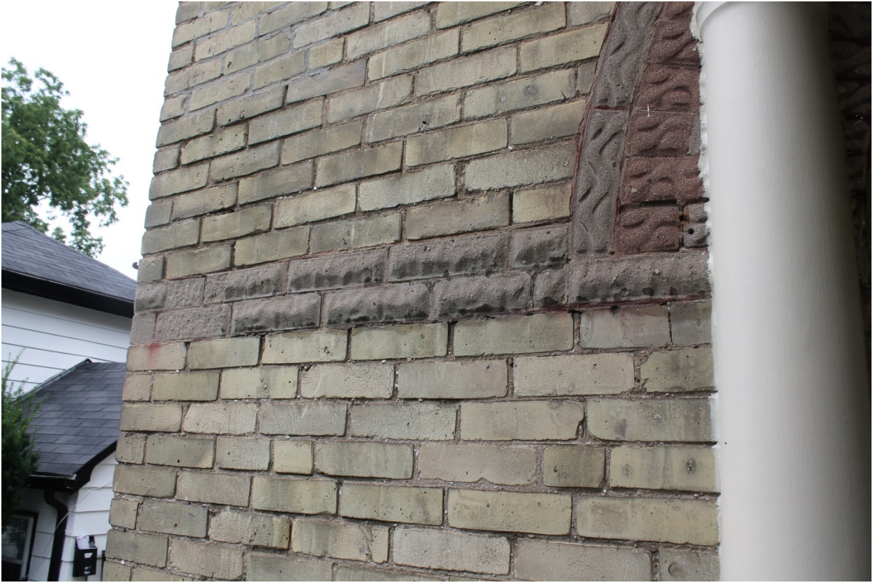
Image 7: Photograph showing buff brick material, rusticated brick string course details and vermiculated voussoirs.
