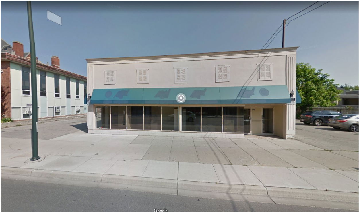
Figure 1: Structure at 496 Dundas Street, facing north.
