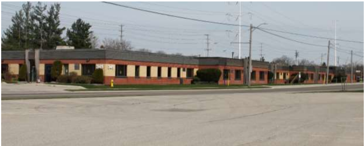
Figure 1: 335-385 Saskatoon Street (West Side) Looking North
