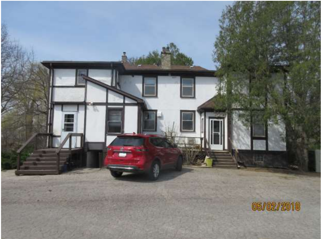
Image 9: Rear (east) façade of the house located at 2154 Richmond Street.
