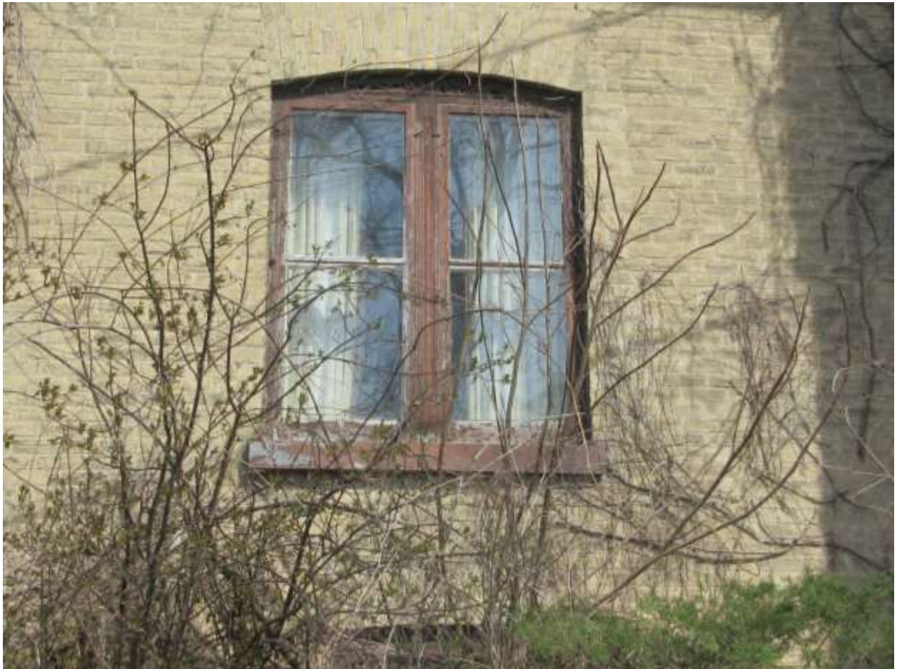
Image 7: Detail of the floral-motif piercework in the wood trim of the window opening on the south façade of the house located at 2154 Richmond Street.
