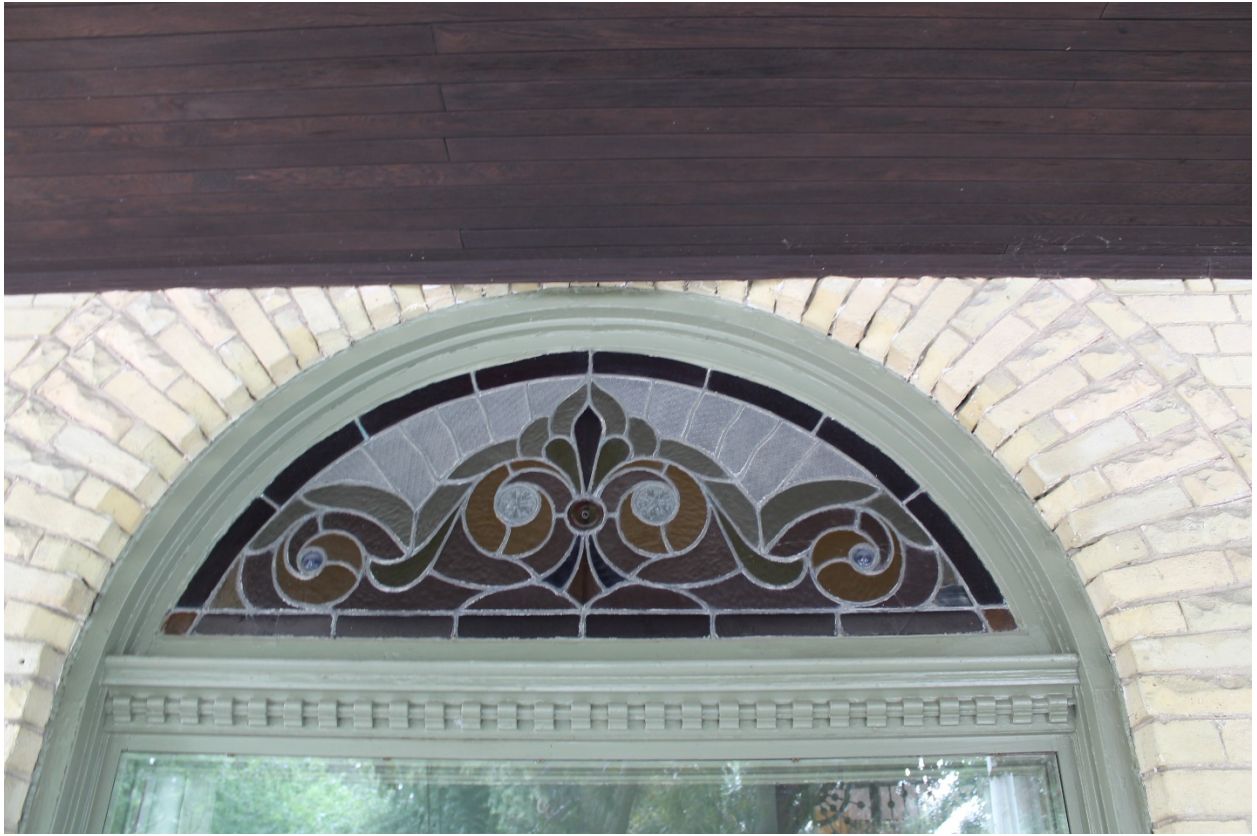
Image 5: Detail showing the heavy trim of the front window and arched stained glass window.
