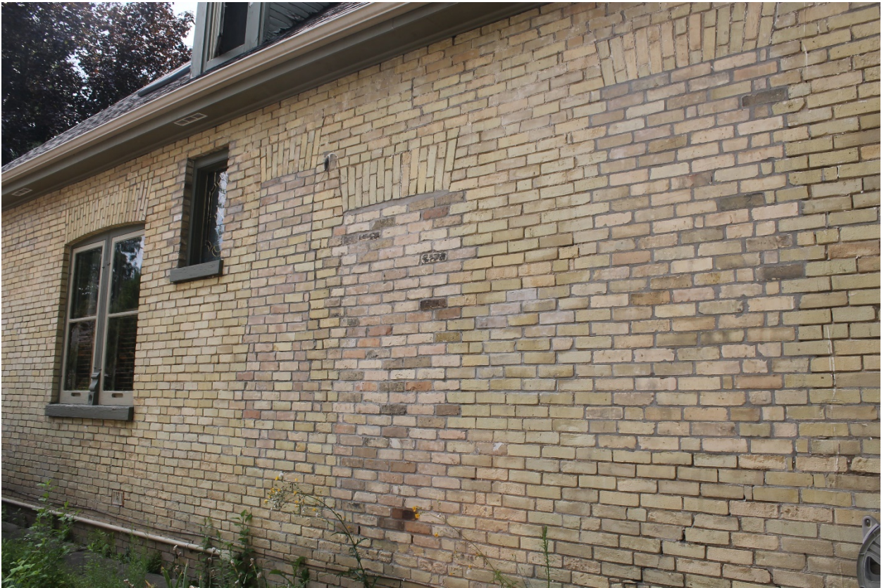
Image 14: Photograph of the east facade of the dwelling showing the remnants of former window openings and the existing windows.
