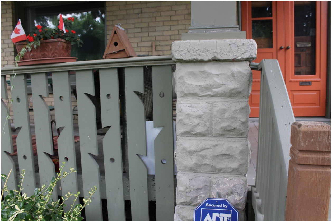
Image 8: Porch details showing rusticated concrete block plinths, wood posts, and railing system.
