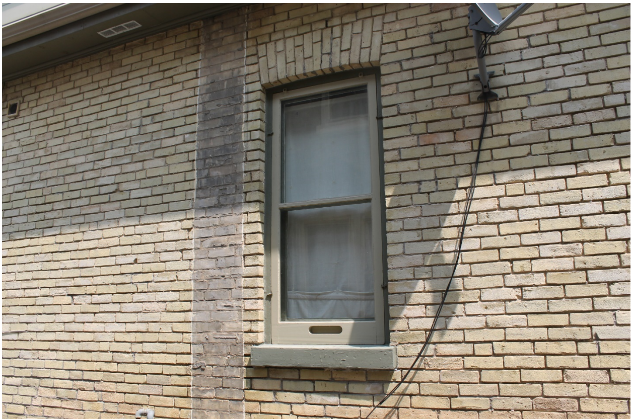
Image 12: Photograph showing double-hung wood window on the west facade of the house, with brick voussoirs and wood sill. Note, the "ghosting" of a former chimney is visible on this wall.
