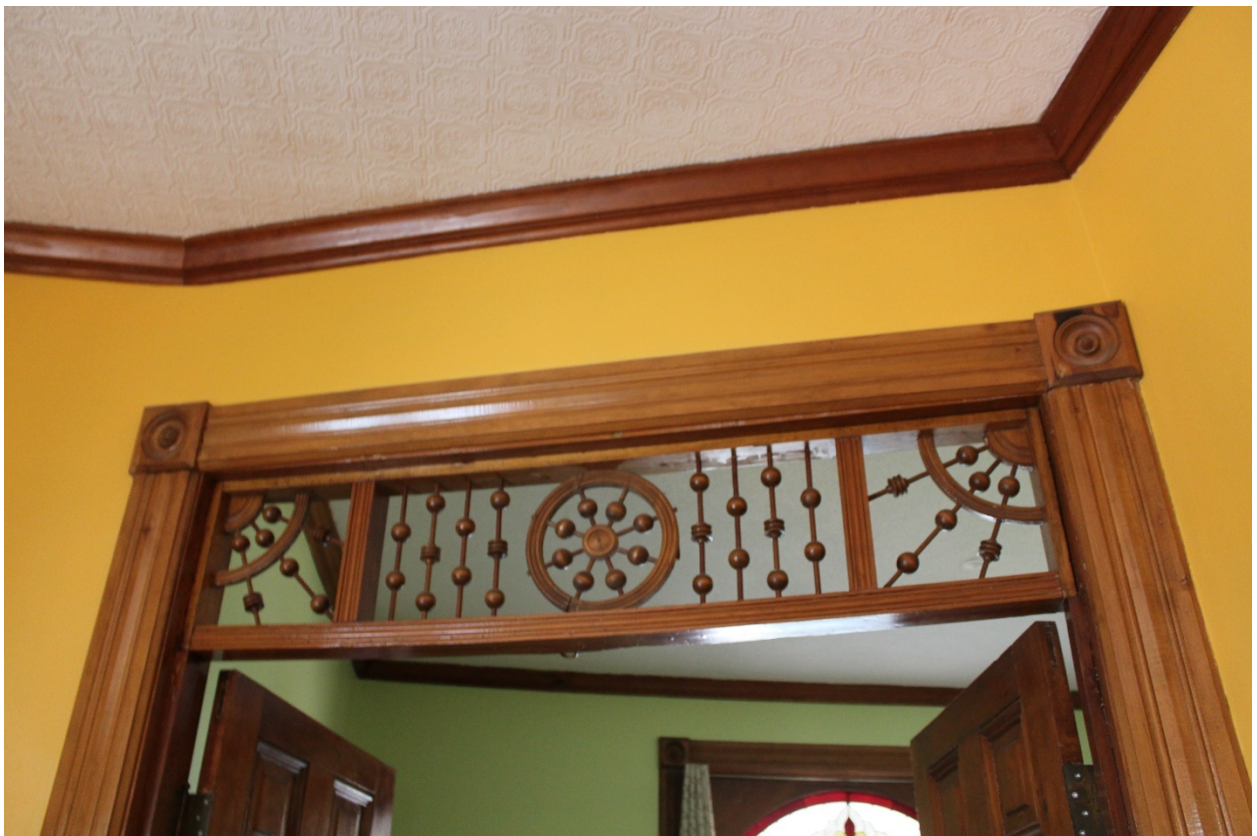
Image 18: Detail showing interior decorative spandrels with beaded design found on the interior of the dwelling.
