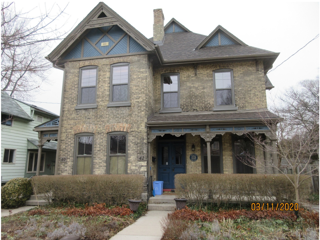
Image 7: Photograph of the properties at 40 & 42 Askin Street on March 11, 2020, showing the replacement windows installed.
