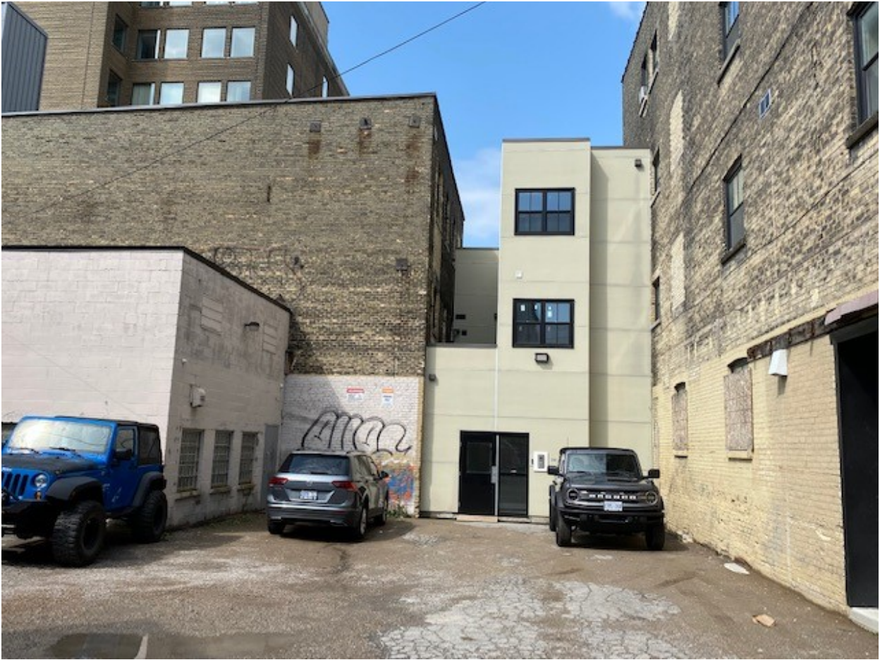
Image 3: View of addition linking front and rear building portions on the property (July 29, 2021)
