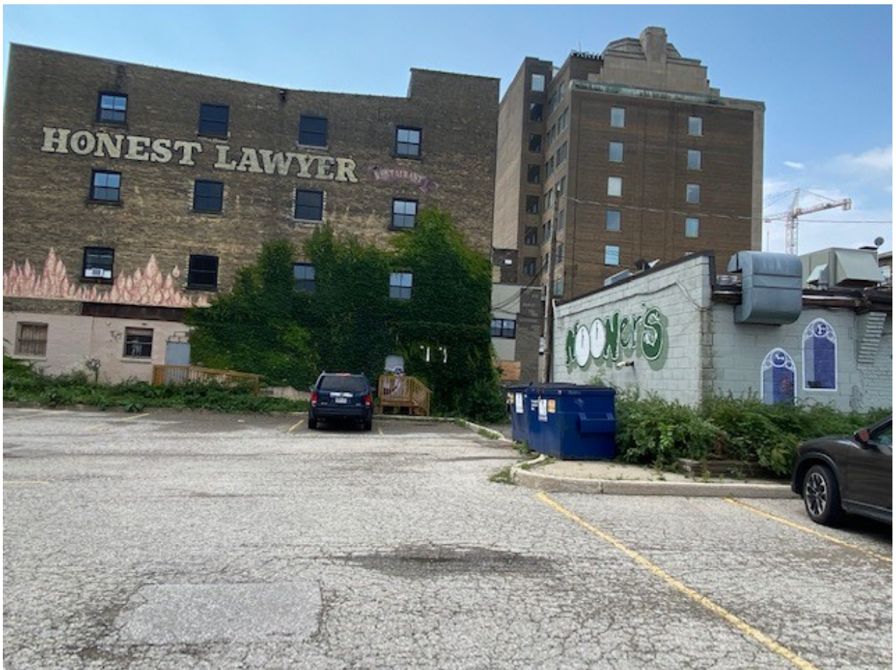
Image 2: View of rear portion of building facing parking lot (July 29, 2021)
