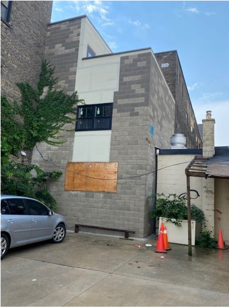
Image 5: View of north facing elevation of unfinished portion of addition (July 29, 2021)
