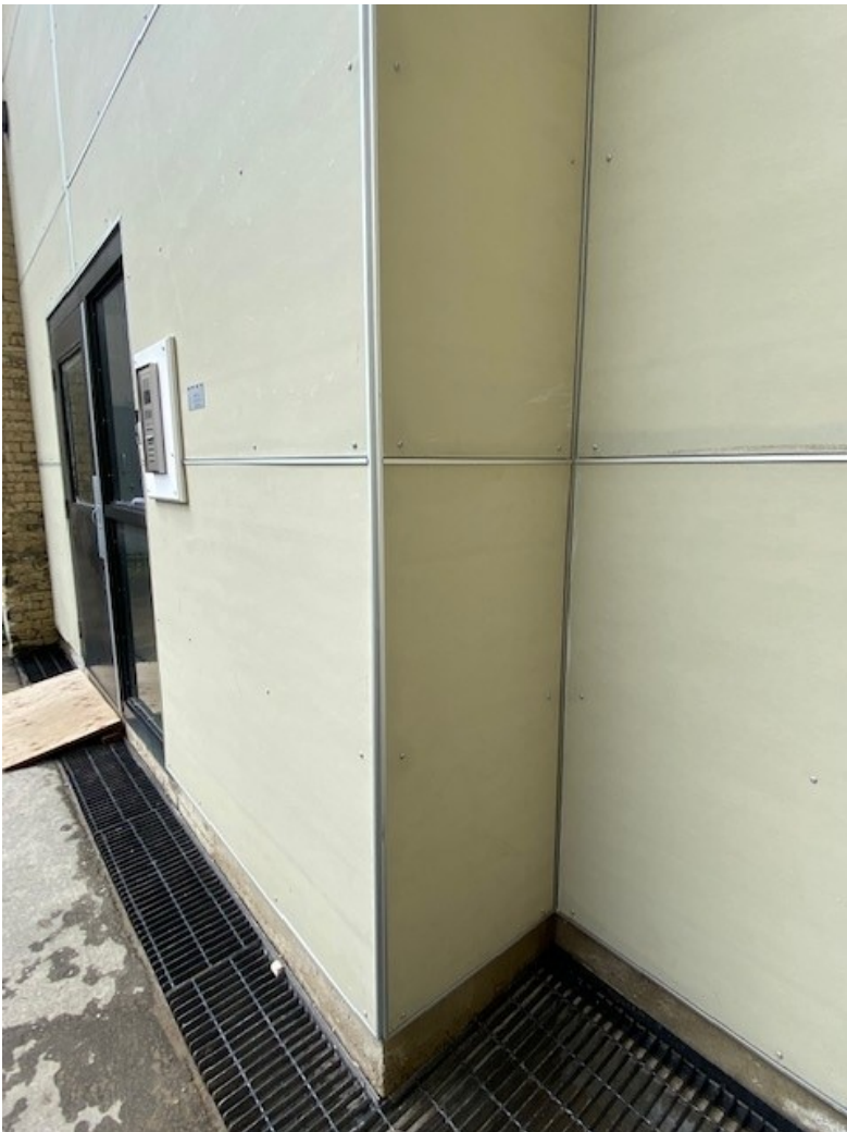
Image 6: Detailed view of cladding material (July 29, 2021)
