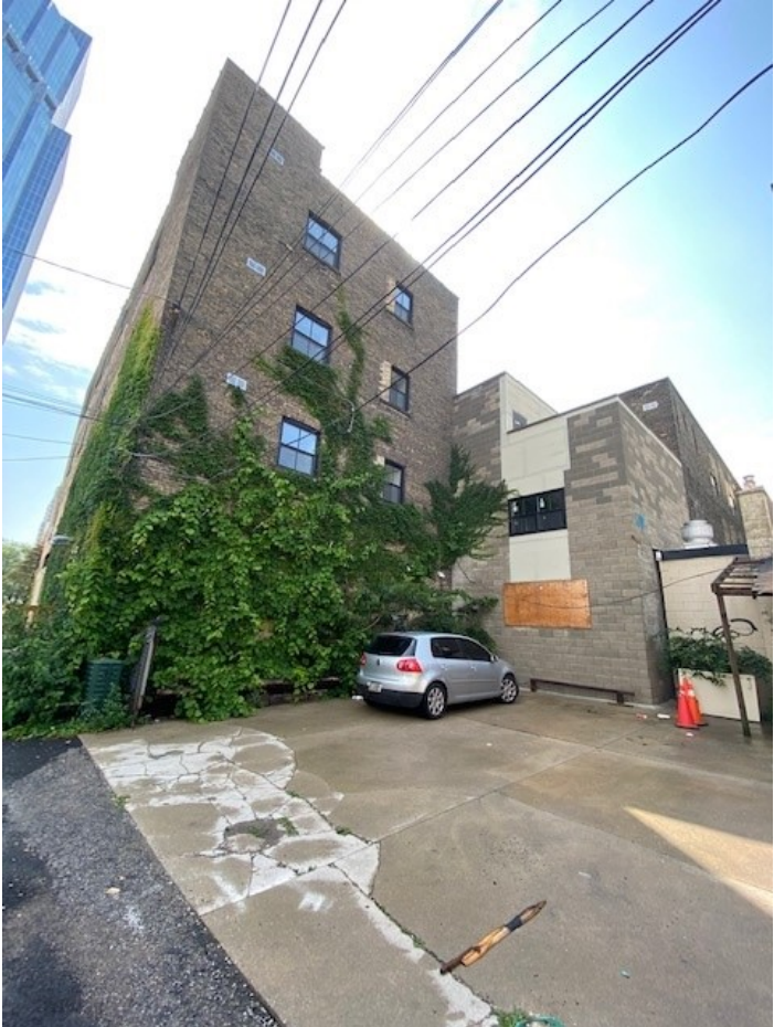
Image 4: View of rear portion of existing building facing parking lot and new addition, seen with unfinished cladding (July 29, 2021)
